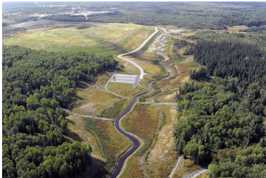
Figure 4.2 : Restored Area along the Turcotte Creek on the Barvue's tailing site (source: MERN Web Site, 2018)
