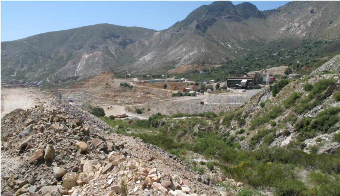
Figure 5.1 View Looking East, showing Aranzazu Processing Plant, Administration Area, Security Pit, and Historic Workings
