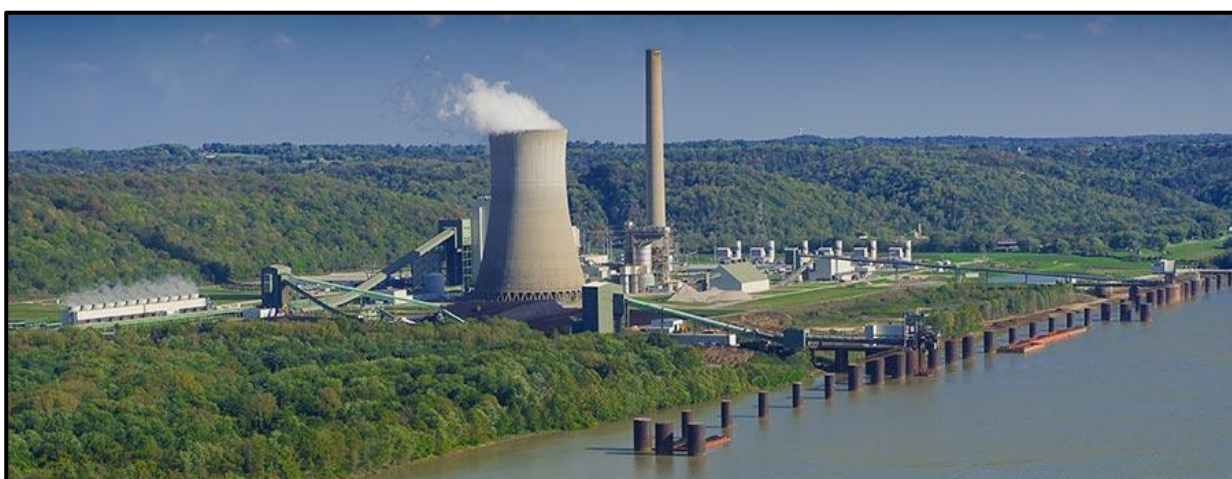
Figure 8: LG&E and KU's Trimble County Power Plant on the Ohio River
