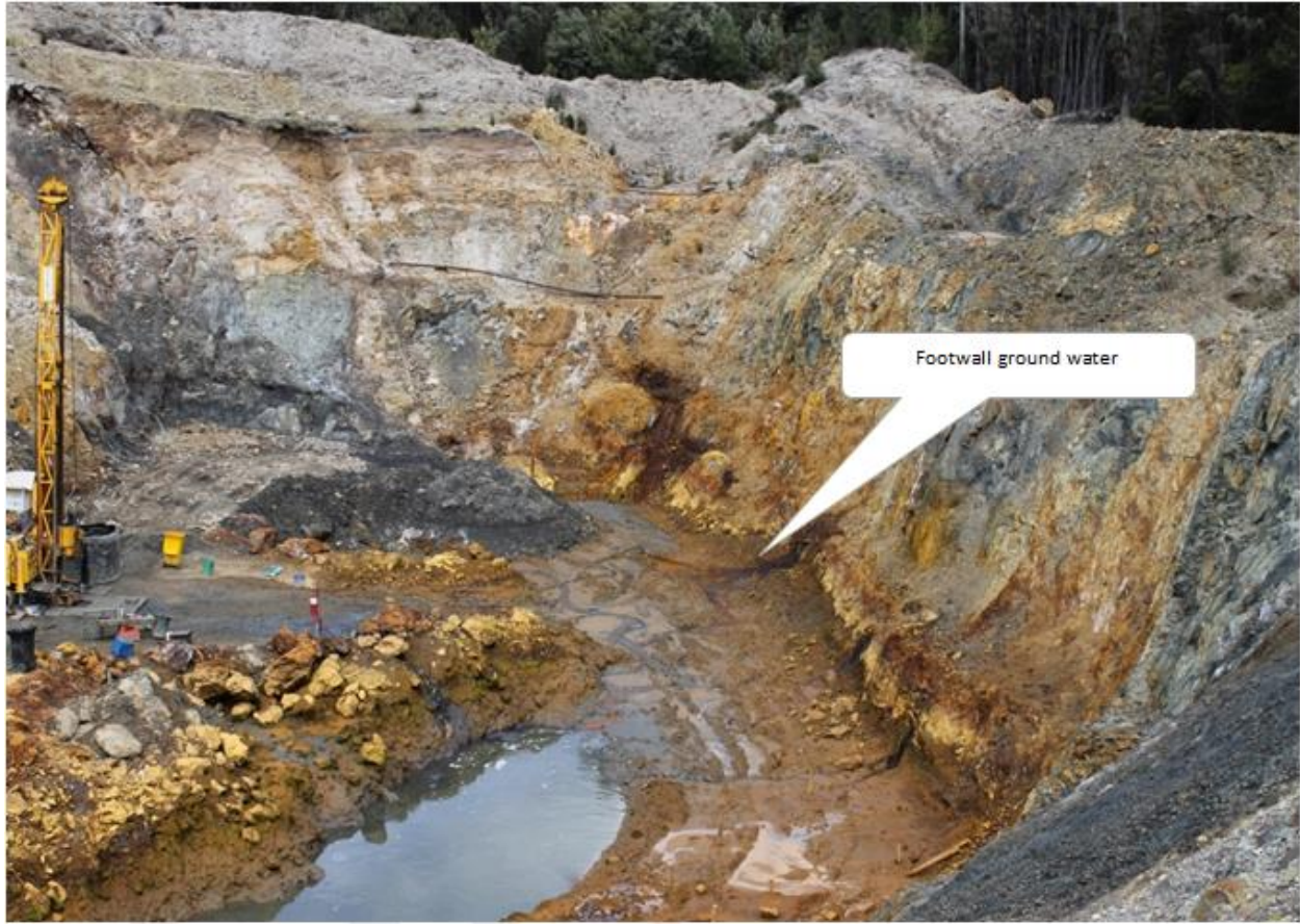
Plate 6.1 - Open Pit at GEM looking south with groundwater seepage highlighted
