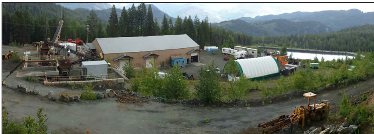
Figure 17.1 Mill Building and Site Area
