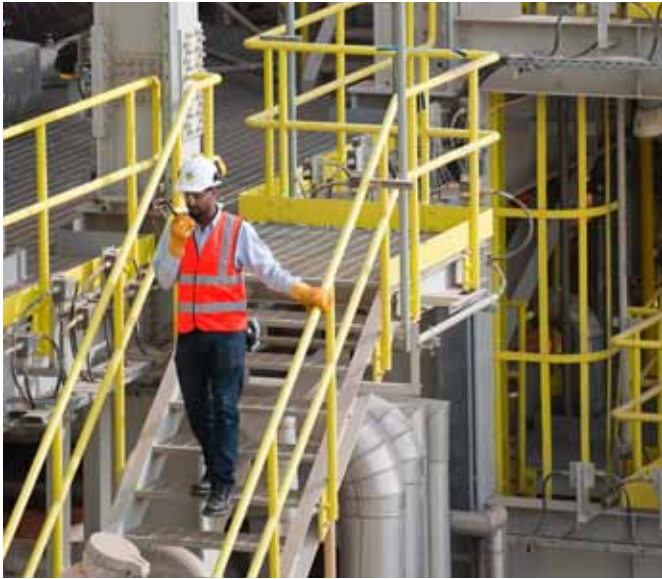
Inspection of the phosphoric acid plant at Ras Al-Khair
