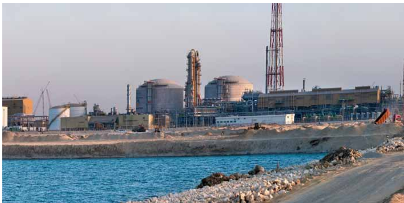
Phosphate complex at Ras Al Khair
