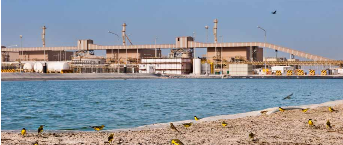
Water retention reservoir at Ras Al-Khair
