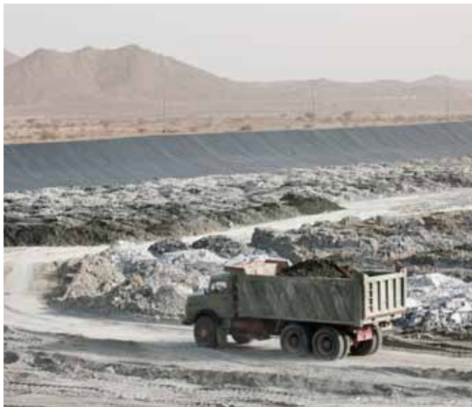
Tailings dam lining at Mahad Ad Dahab
