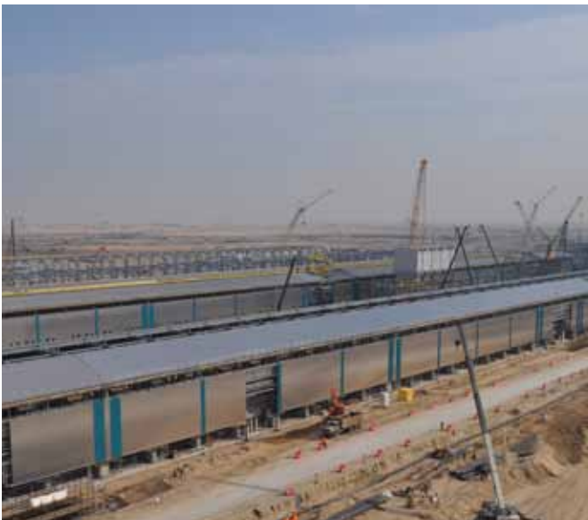
Progress on the aluminium potlines
