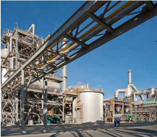
The phosphate plant at Ras Al-Khair
