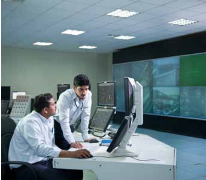
Information technology control centre
