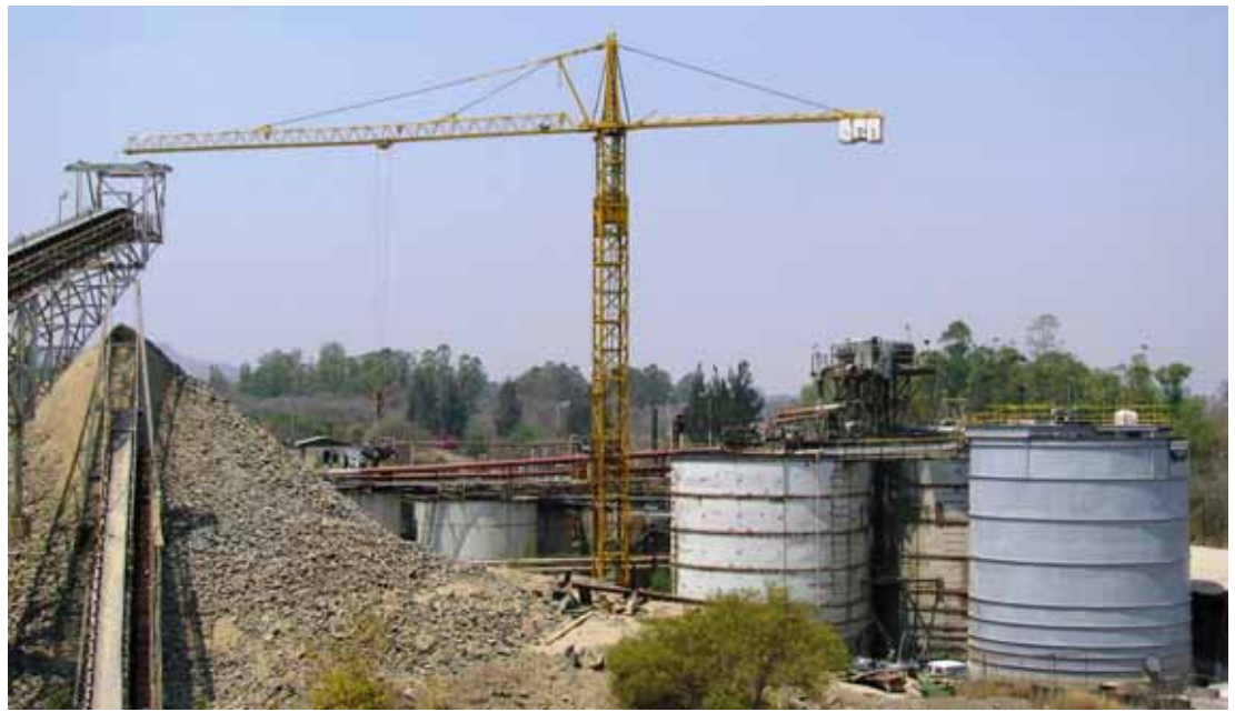
Figure 84. CIL tanks and ore stockpile
