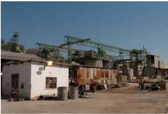
Figure 63. Blanket gold plant
