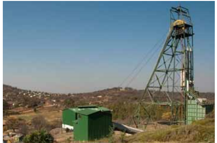
Figure 59. Blanket No 4 shaft
