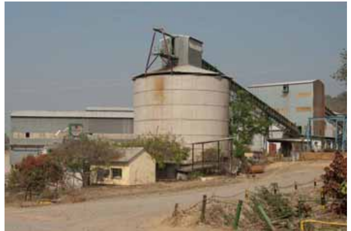
Figure 70. Surface infrastructure at Renco mine
