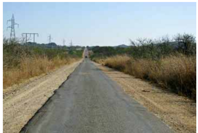
Figure 4. Secondary narrow tarred road near Gwanda
