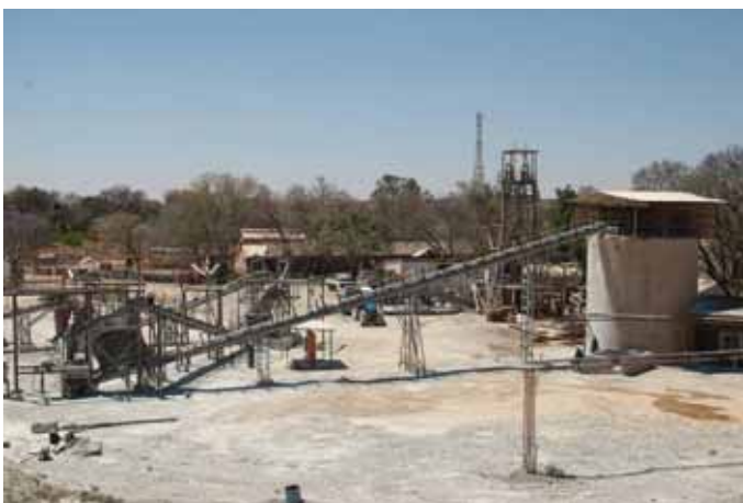
Figure 47. Turk mine surface infrastructure
