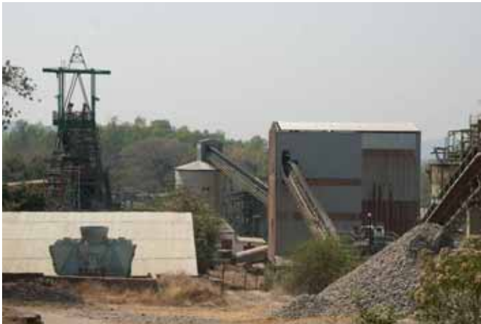
Figure 69. Surface infrastructure at Renco mine
