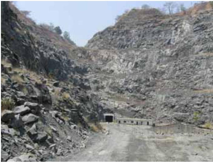
Figure 76. Entry to underground workings
