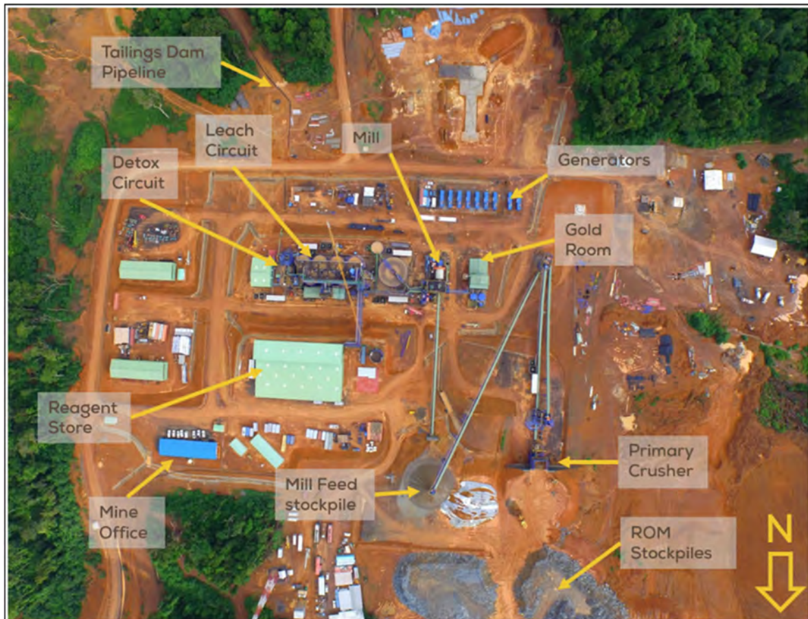
Figure 5-2: New Liberty site infrastructure Source: www.avesoro.com , 2019
