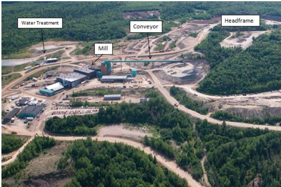
FIGURE 18-1 AERIAL VIEW OF CARIBOU SITE INFRASTRUCTURE
