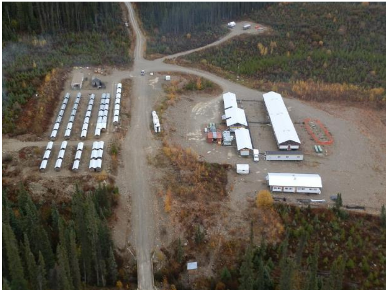
Figure 4-2: Aerial View of the Akie Camp
