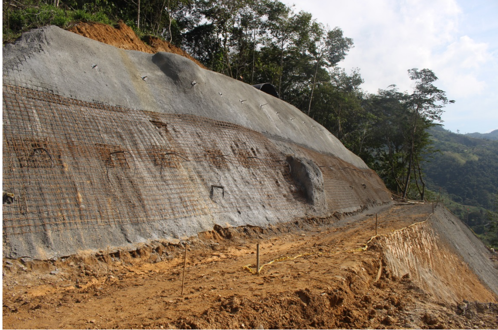
Photo 7: Slope Stabilization in Plant Site
