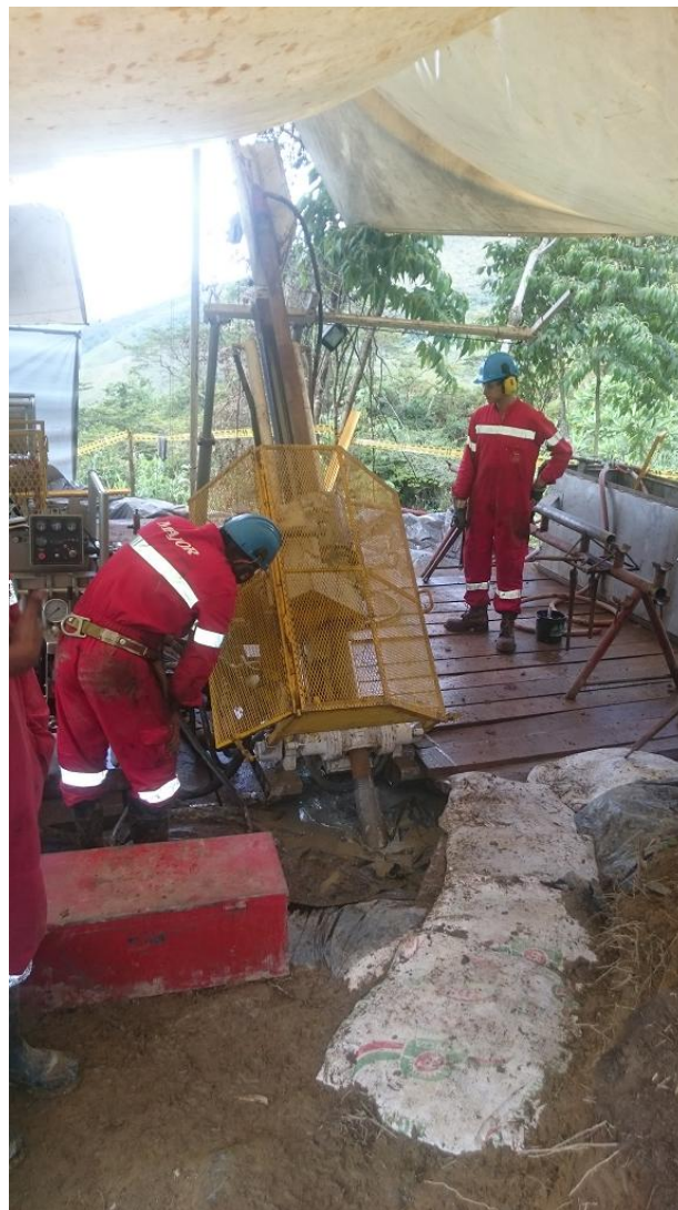
Photo 4: Drill Rig – Guayabito Sur Area (2016)
