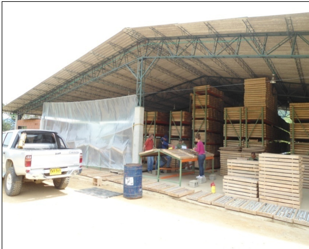
Photo 2: Core Warehouse at the Cisneros Project
