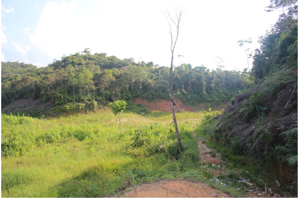
Photo 8: El Hormiguero Tailing Storage Facilities Area
