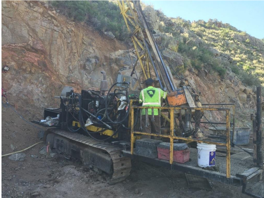
Figure 12.1: Godbe Drill Set-Up of Hole WG-16-34
