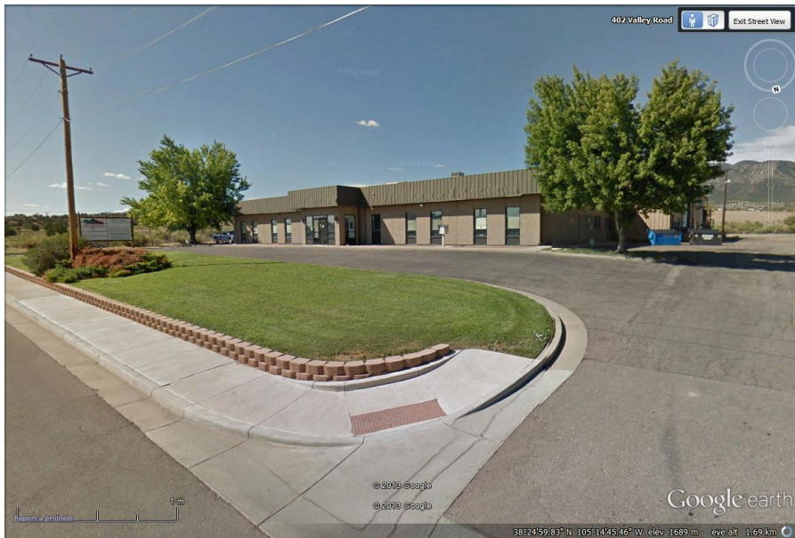
Figure 12.15: Location of 2013 Zephyr Core Logging Facility in Cañon City, CO
