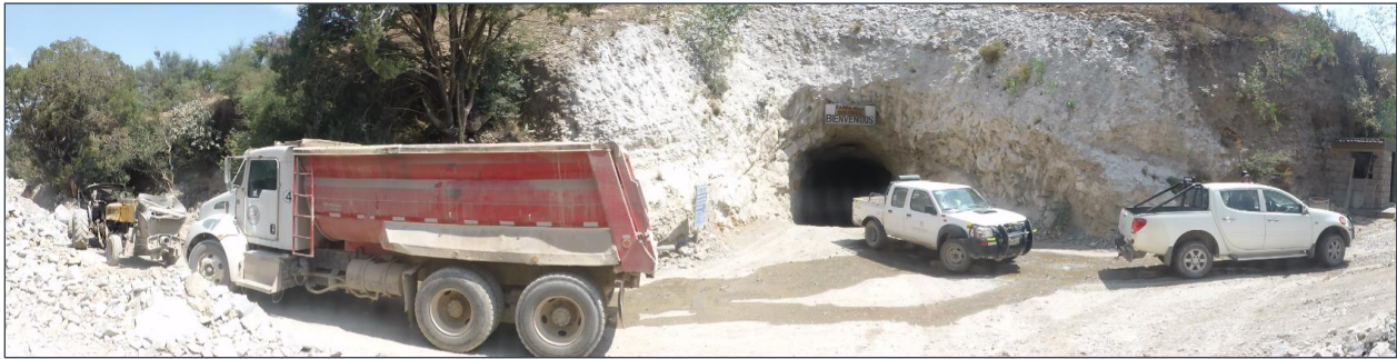
Figure 16-16: Dolores Mine Portal
