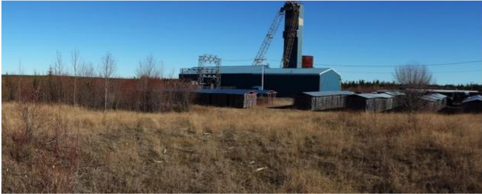
Figure 18.4 View of the Office/Dry/Hoist house Complex from the Northwest
