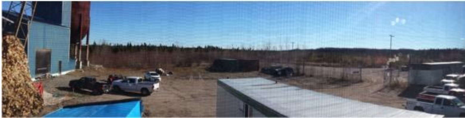
Figure 18.1 View from Offices South to Proposed Pit Location and West (panorama)
