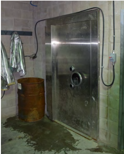
Figure 18-17 - Gold Room Vault
