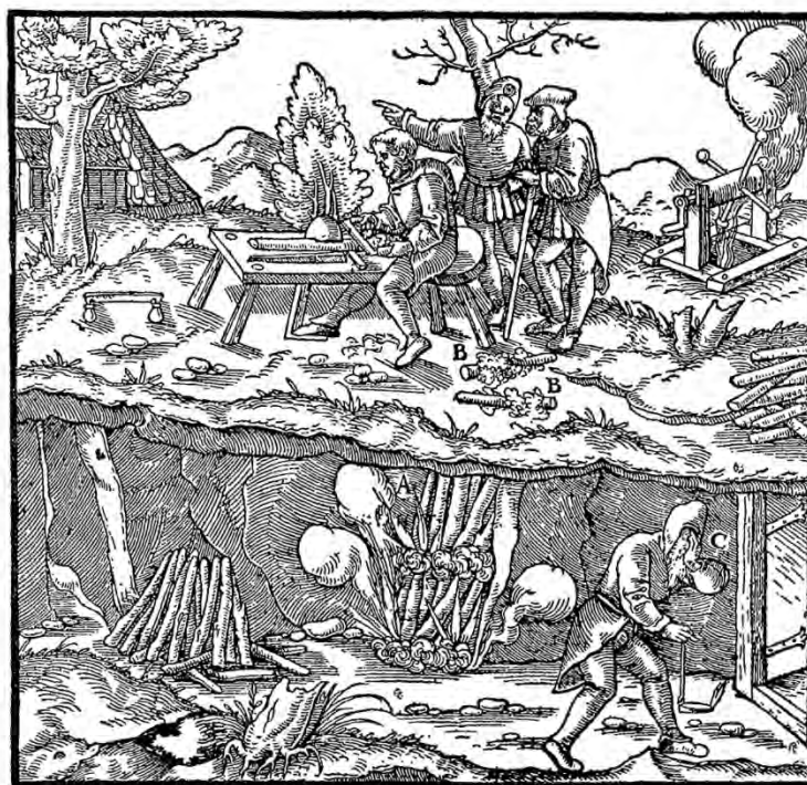
A—KINDLED LOGS. B—STICKS SHAVED DOWN FAN-SHAPED. C—TUNNEL.
