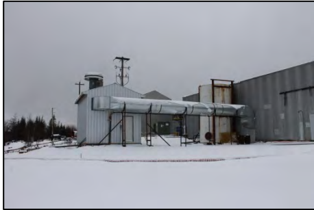
Figure 18-5 - Compressor House & Rear of Mill
