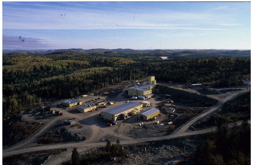
Mill – Mineral processing complex Looking northeast
