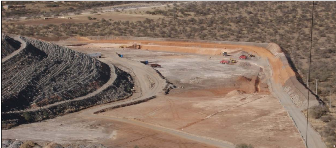
Figure 71: Tailings facility expansion under construction (SRK, February 2017)
