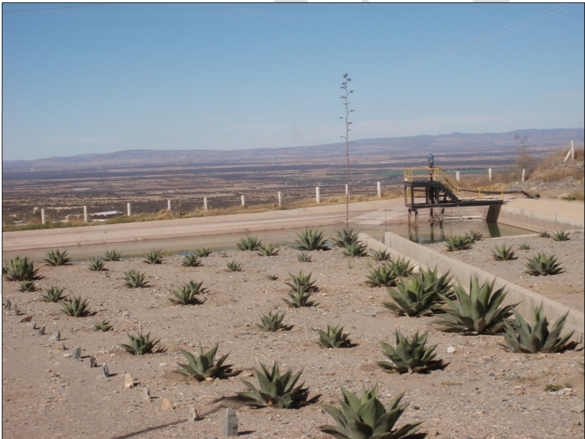
Figure 73: Dirty-water catchment below processing plant (SRK 2017)
