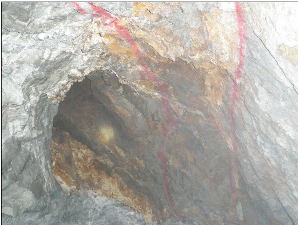
Figure 47: Good Rockmass Quality in Oxide MCF Stope at Quebradillas (SRK 2017)
