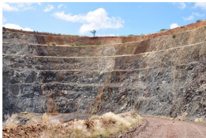
Figure 7-3 Photograph of the eastern wall of the Tau open pit. Bench heights are 15m
