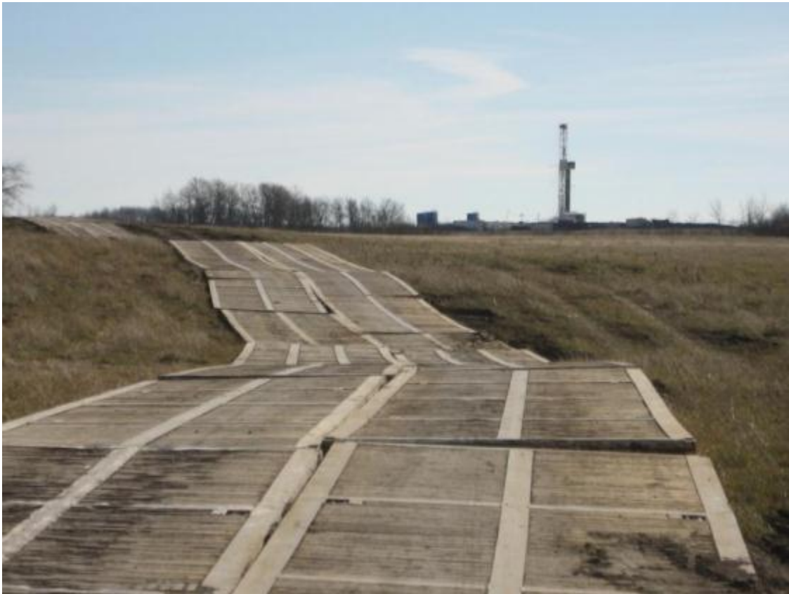
Figure 5-1: General topographic features of the area along the matted 07-02-027-15W2 lease access road. Drill rig ensign 25 is shown in the distance. (Source: North Rim)
