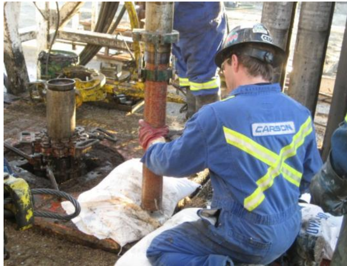
Figure 10-2: Blackie’s Coring Services Performing Core Retrieval.
