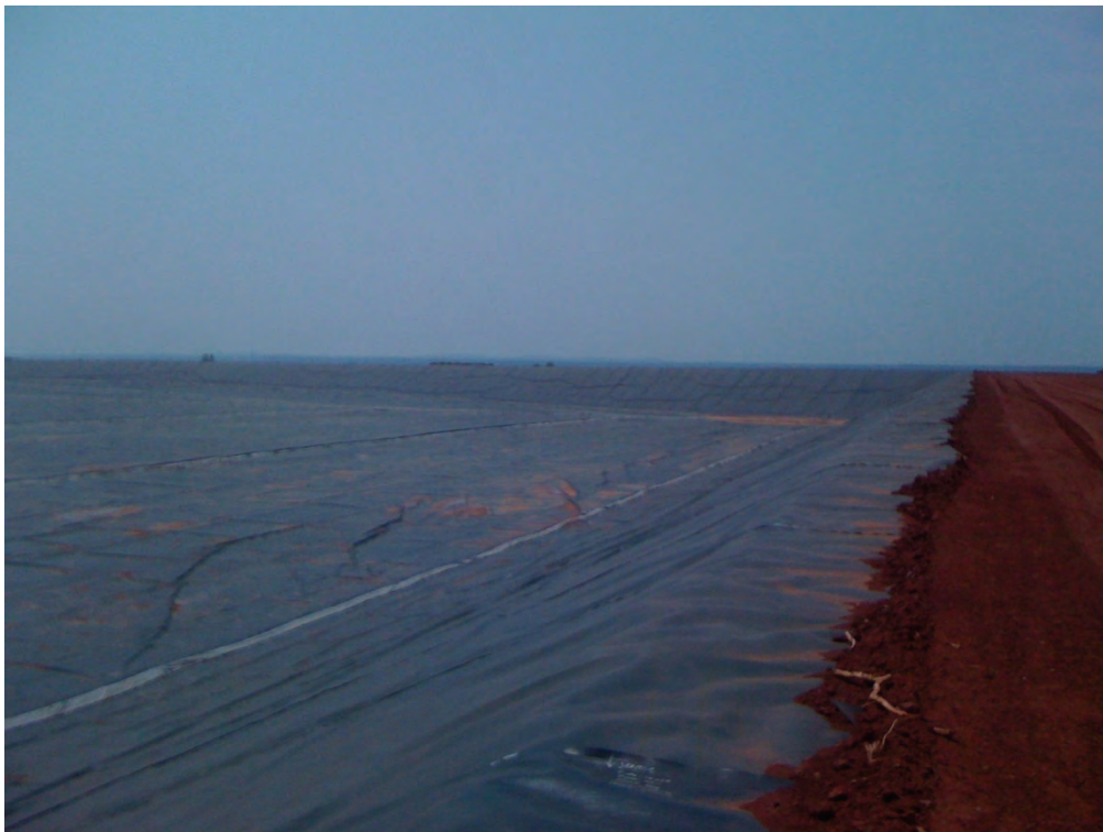
Figure 67: Basin of Mutanda Tailings Dam as seen from the western embankment
