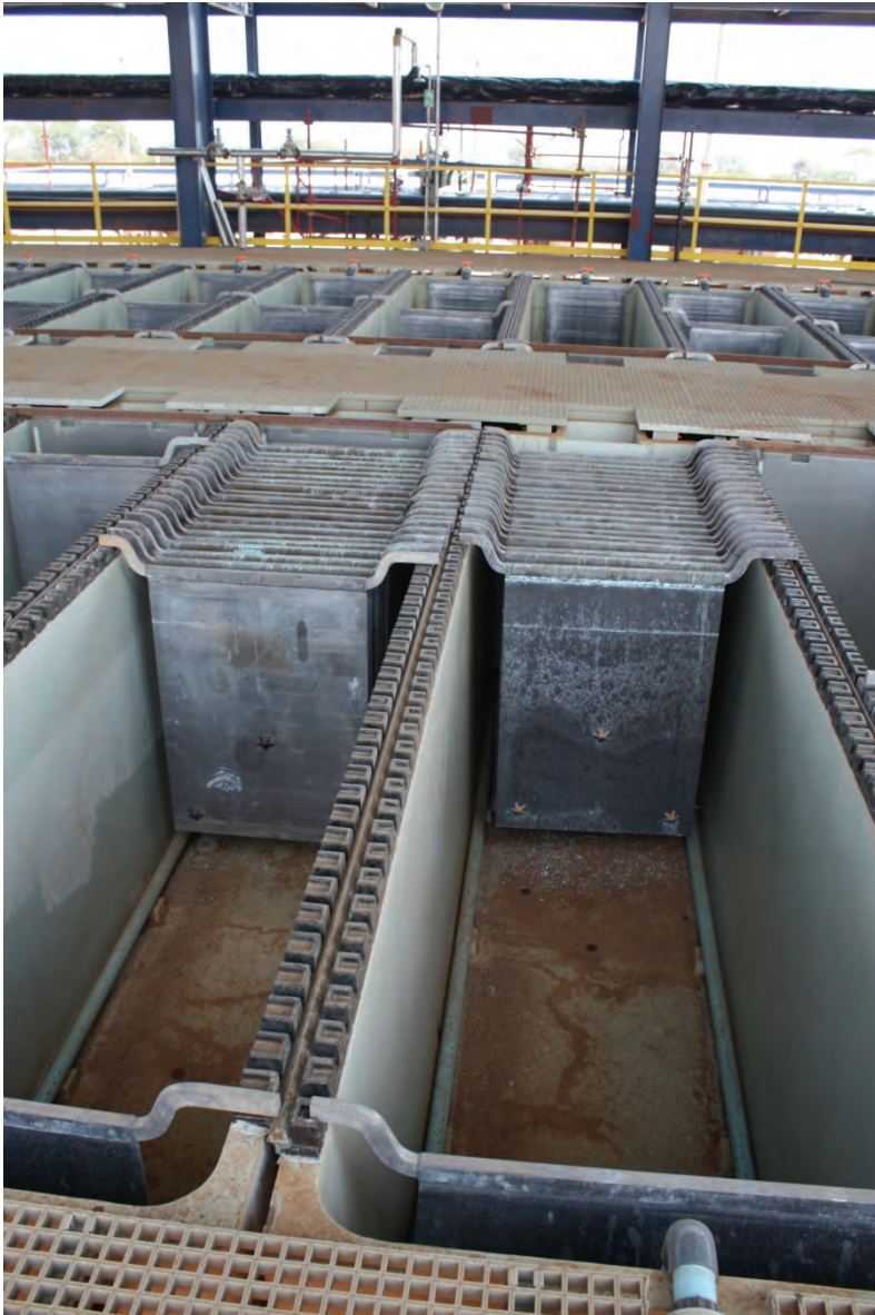
Figure 60: Lead Anodes being fitted to the Electrowinning Cells during construction
