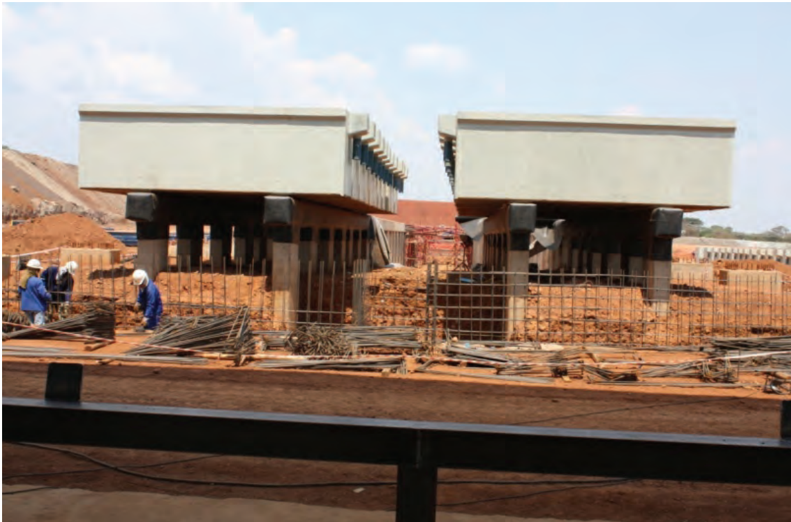
Figure 64: 40 000 tpa Module Electrowinning Cells Already in Position
