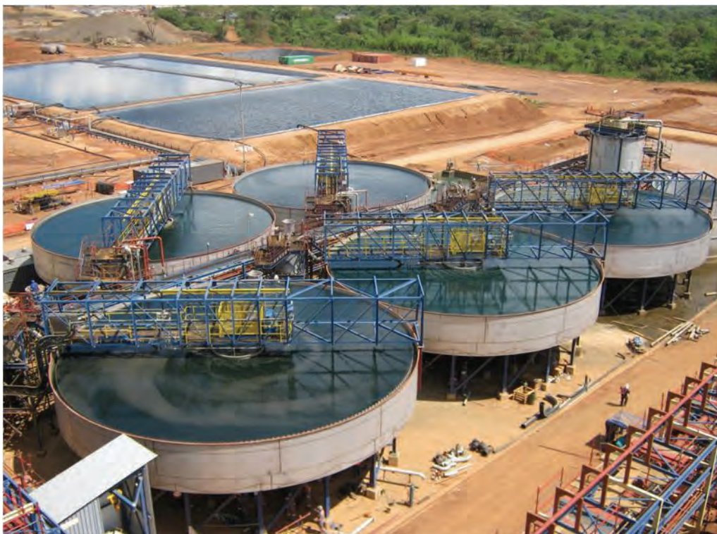
Figure 56: Counter Current Decantation Vessels with PLS ponds in the background
