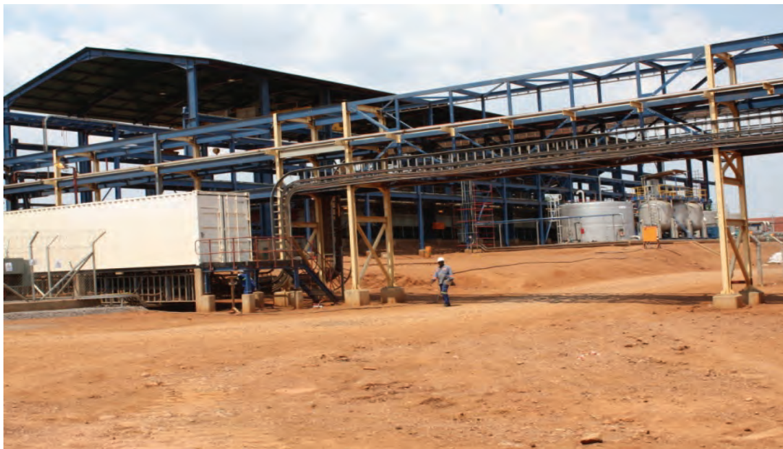
Figure 58: Tank House External
