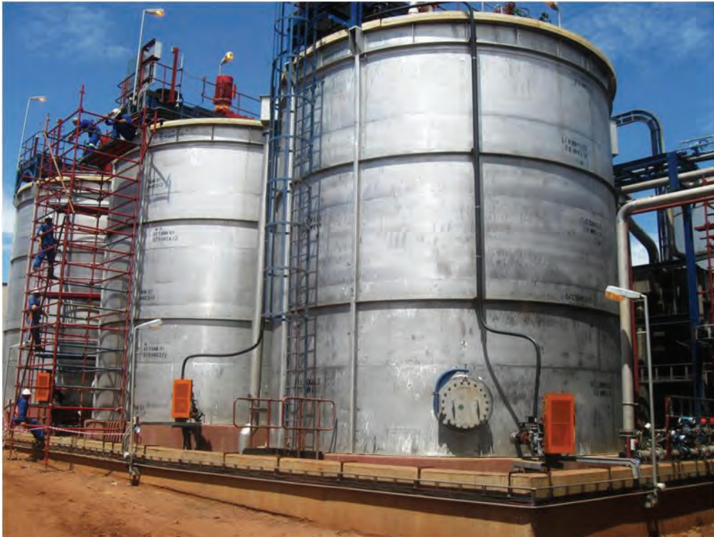
Figure 55: Leach Tanks
