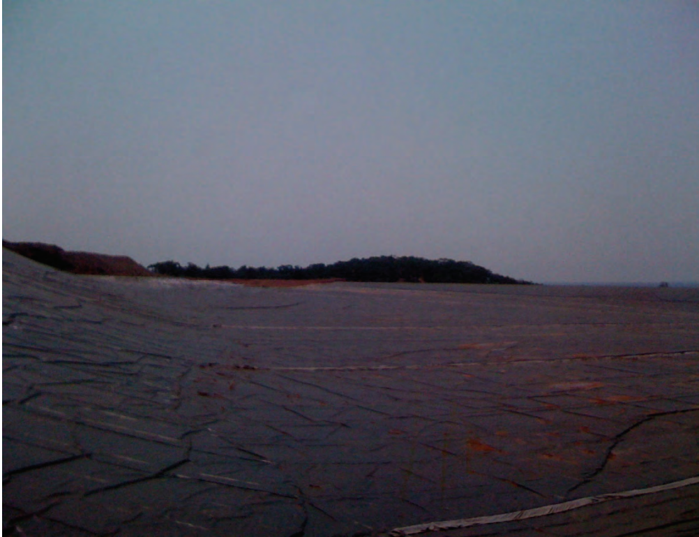
Figure 68: Mutanda Tailings Dam during liner installation
