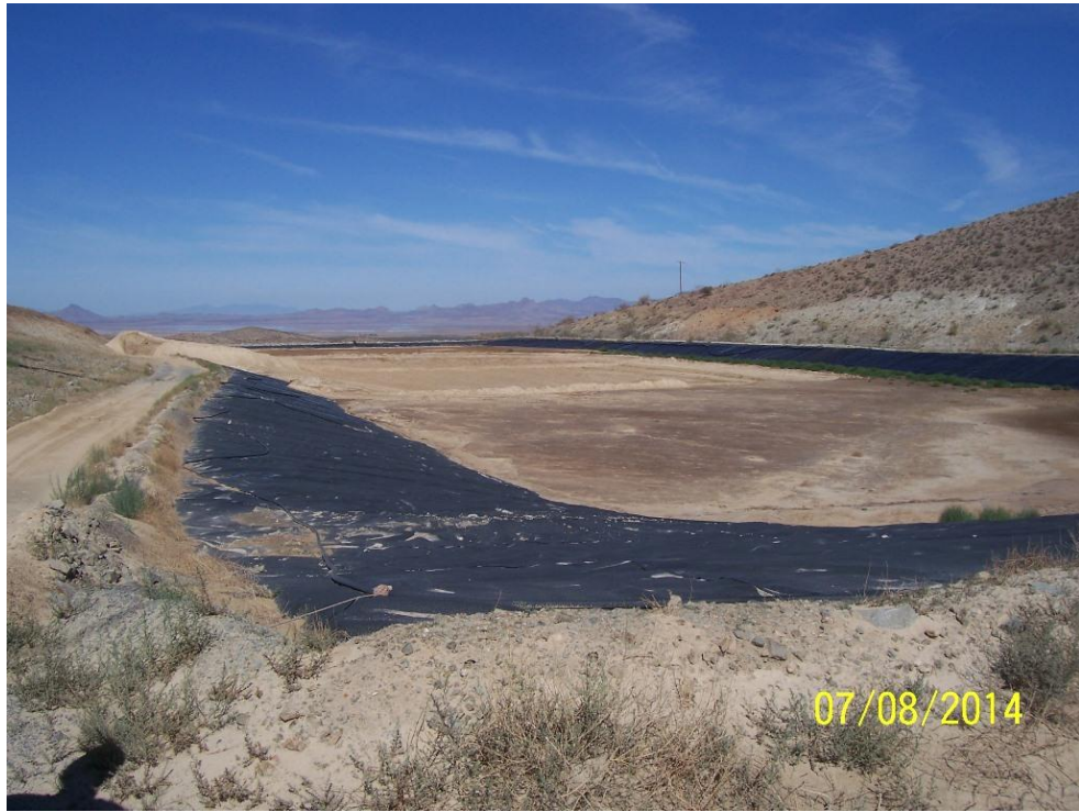
Mill-tailings facility looking west (July 8, 2014)
