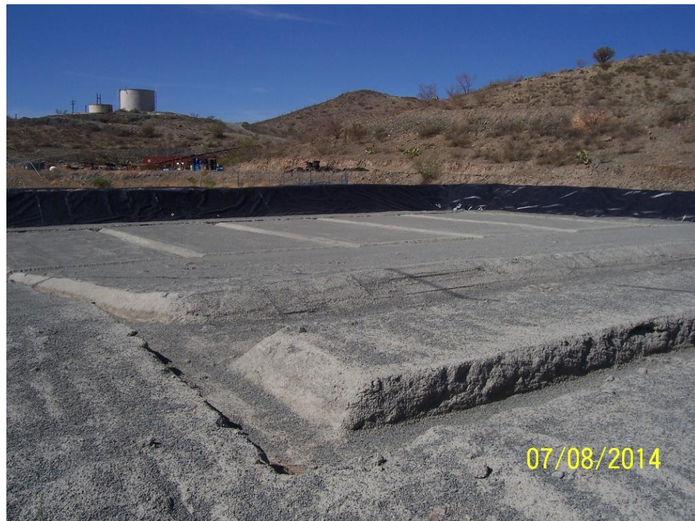
Tailings decant-cell under construction; looking S 25°W (July 8, 2014).
