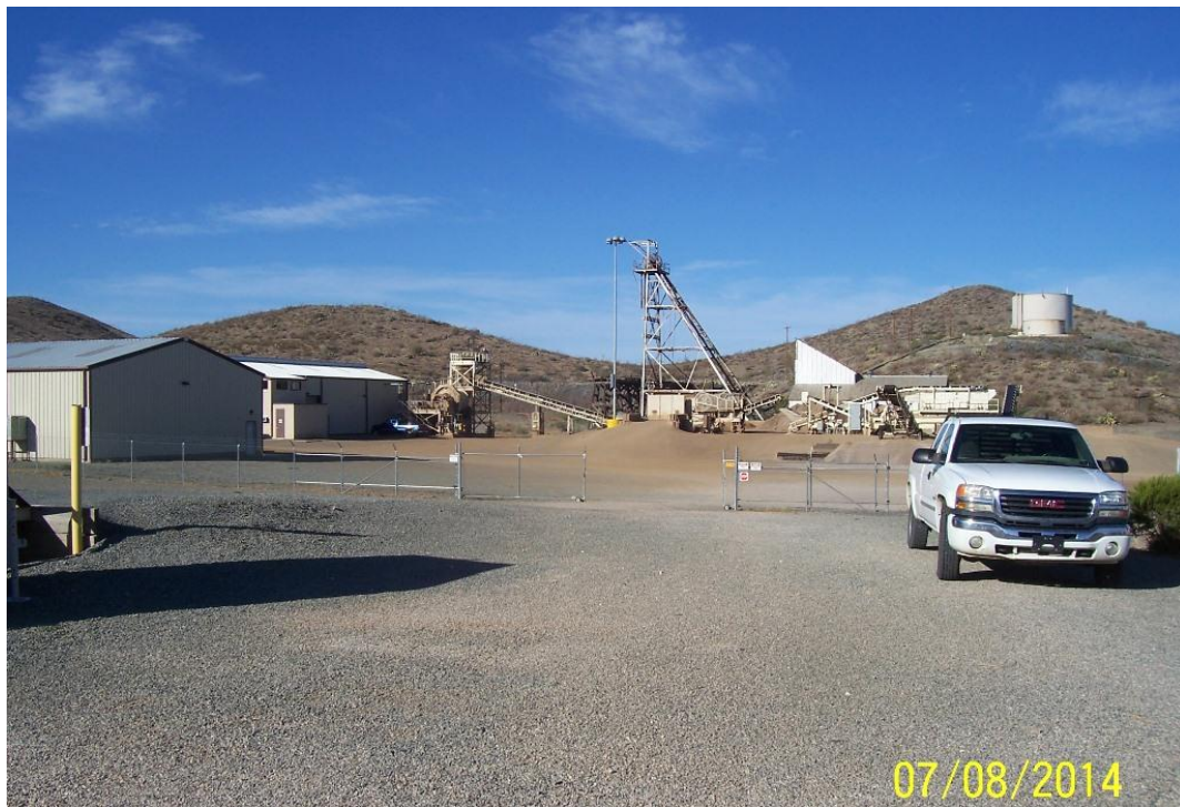
Lordsburg (Banner) millsite; looking S 25°W; the Banner shaft (water source) and old hoist house in center; ball mill, mill building and shop to left; crushing plant and mill head tank to right.
