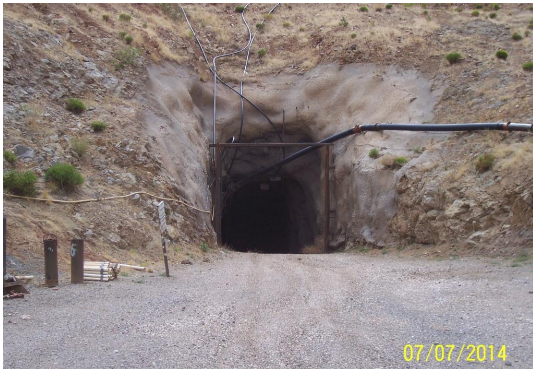
Main decline portal; looking southwest.
