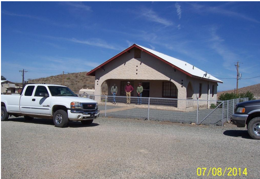
Lordsburg operations office at the millsite; looking west.
