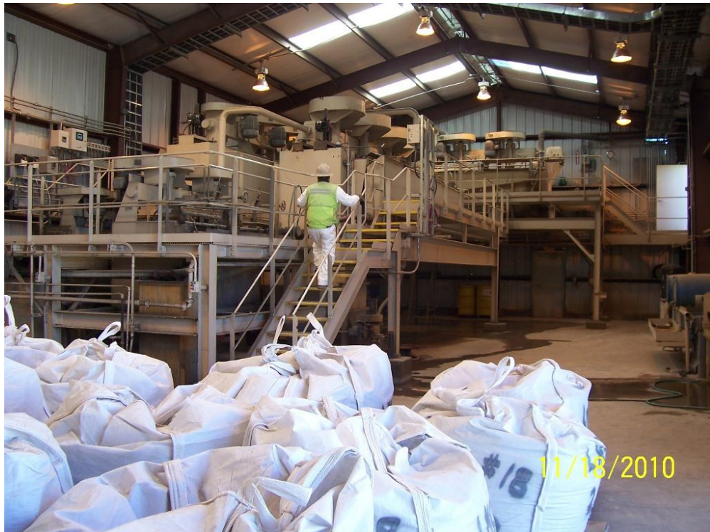
A portion of the flotation section in the mill with bagged concentrate.
