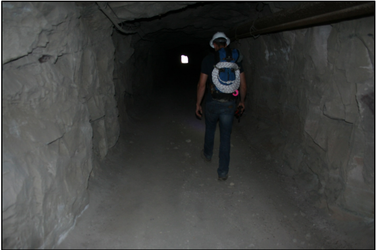
FIGURE 16.3: CONDITION OF BURRO MINE DECLINE
