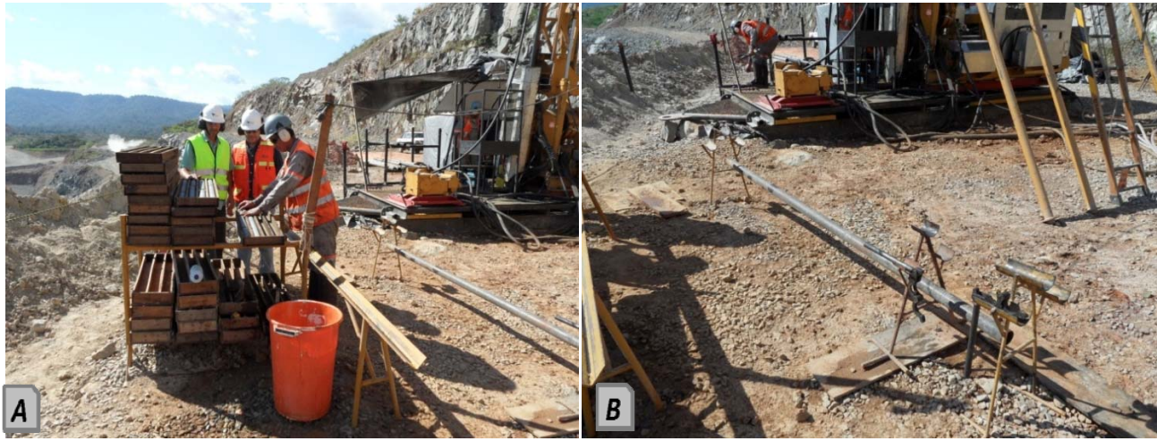
Figure 8-11: A) Core piled up on rig platform waiting to be transported. B) Equipment use for core sampling
