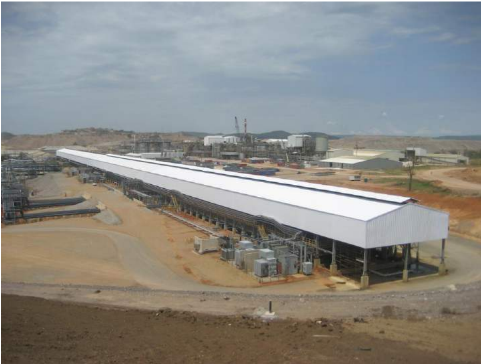
Figure 1-3 Tankhouse Completed as seen in November 2013
