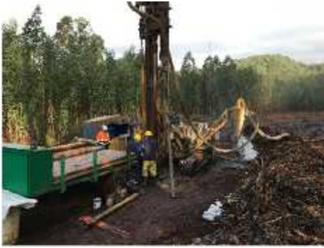
Picture 1 RC drilling on site
