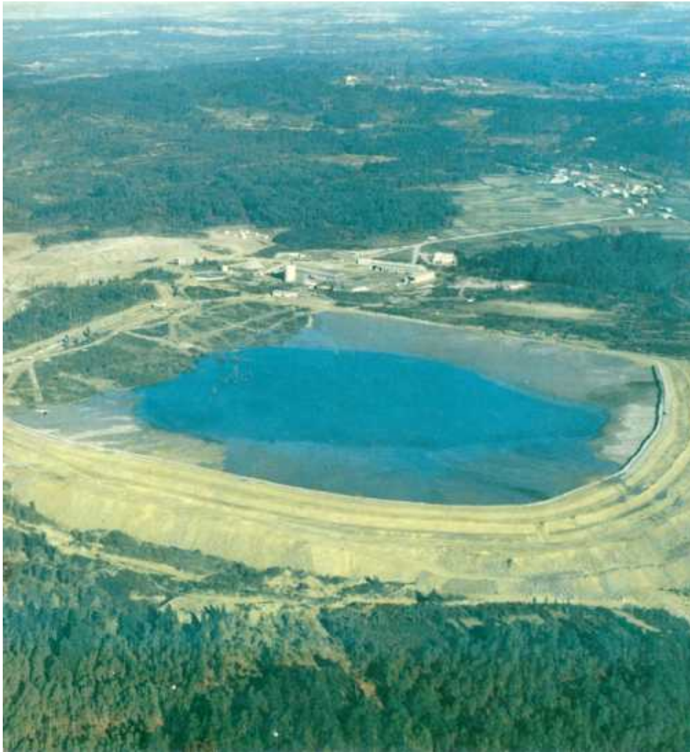
Figure 6.5 – Presa Nueva Tailing Storage Facility in 1986 (Atalaya 2017)
