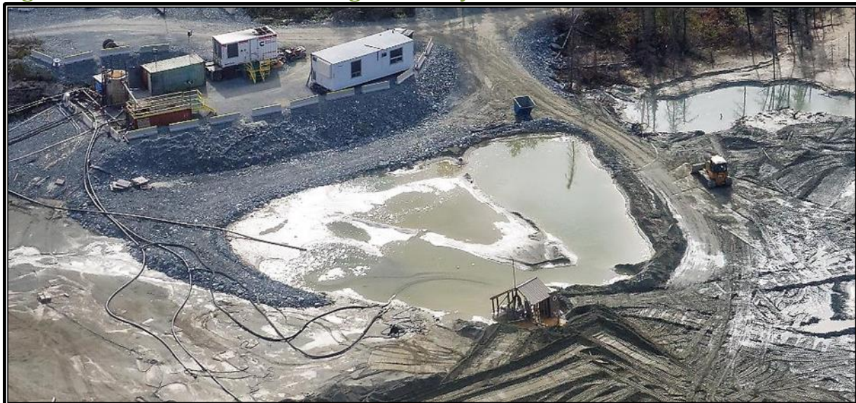
Figure 24-10 Aerial View of Tailings Recovery Site
