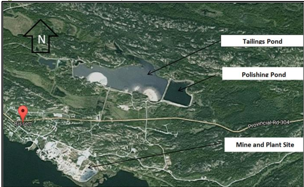
Figure 4-5 Aerial View of the Mine, Plant Site and TMA
