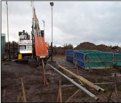
Figure 10-1. Drill Set-Up – Hole VS002
