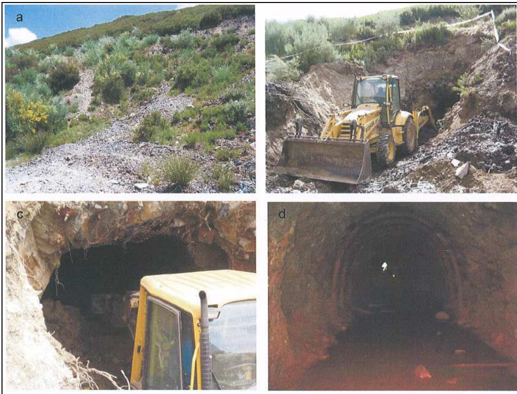
Figure 6-3. Re-establishing Access to Underground Gallery
