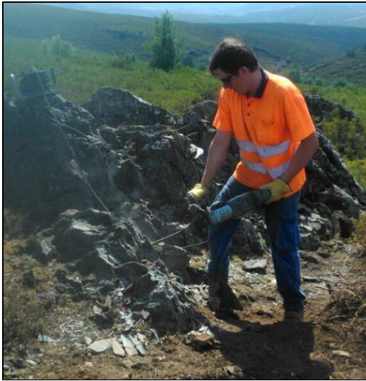
Figure 9-2. Use of Electric Hammer
