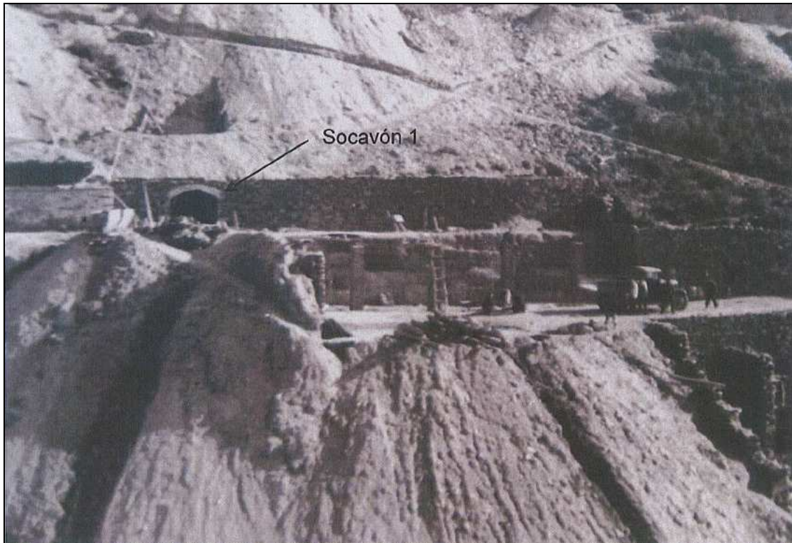
Figure 6-1. Construction of Historical Ore Washing Plant and Gallery Entrance
