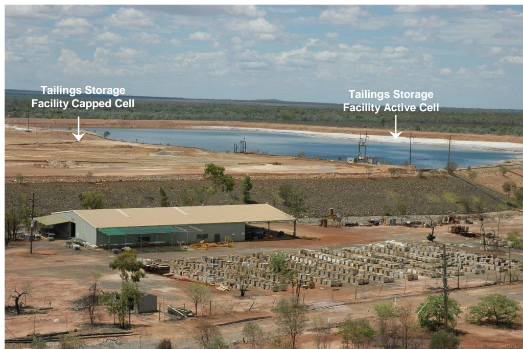
Figure 10 Tailings Storage Facility
