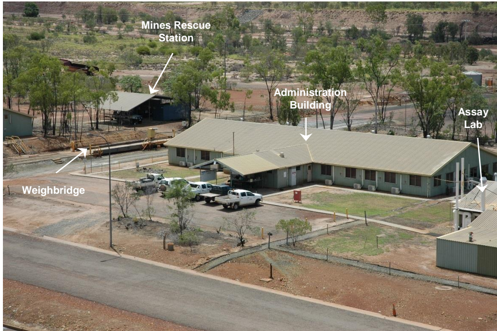
Figure 12 Thalanga Project infrastructure – site entrance, weighbridge, administration office and assay laboratory
