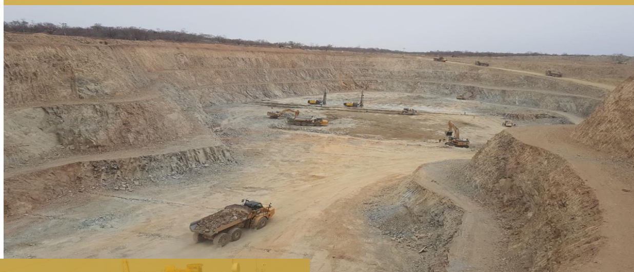
A2NE Open Pit
