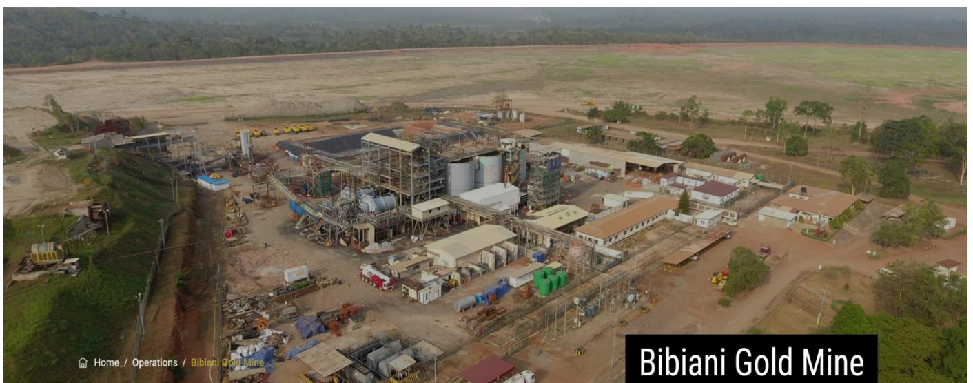
Figure 17-2: View of Bibiani Processing Plant with TSF in Background
