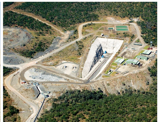
Figure 4. Aerial view of Portal 1 (Ngwarati) Mine
