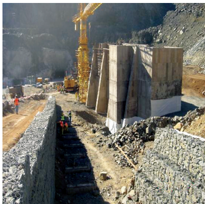
Figure 2. Portal 2 (Rukodzi) Crusher station under construction
