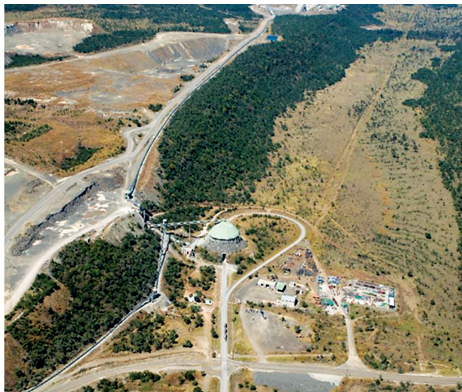
Figure 6. Aerial view of equipment and services common to Portals 1 and 2
