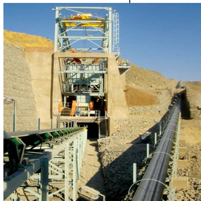
Figure 3. Portal 2 (Rukodzi) Crusher station completed
