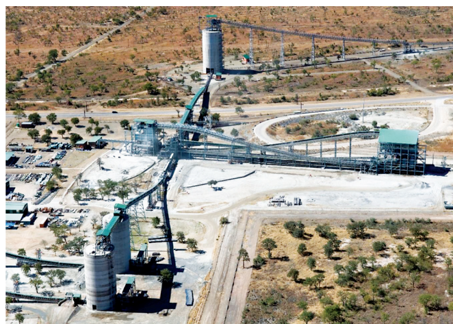
Figure 16. Ngezi Concentrator materials handling
