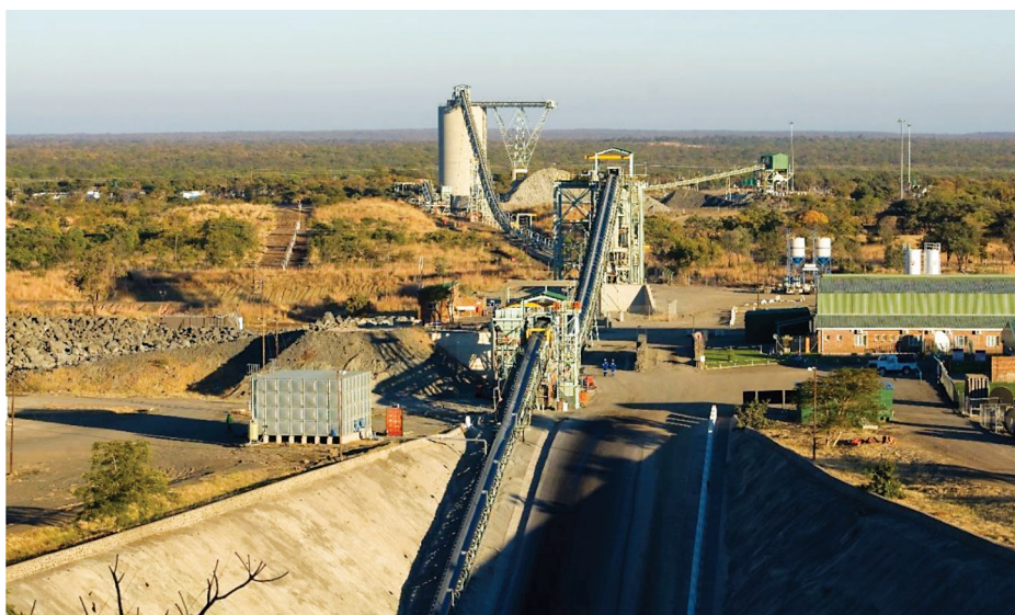
Figure 9. Portal 4 (Bimha Mine)
