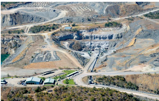
Figure 1. Aerial view of Portal 2 – Rukodzi Mine
