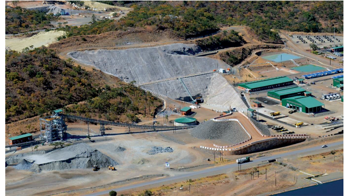
Figure 13. Portal 3 (Mupfuti Mine)
