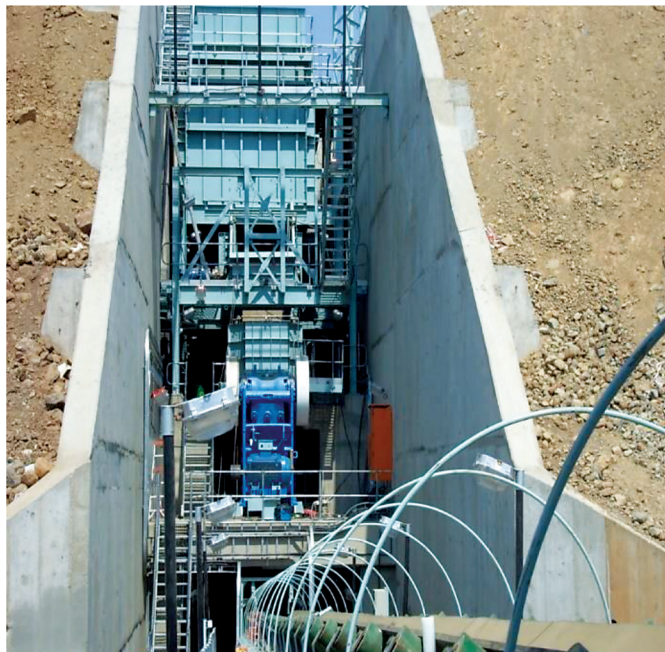
Figure 5. Portal 1 (Ngwarati) Crusher Station
