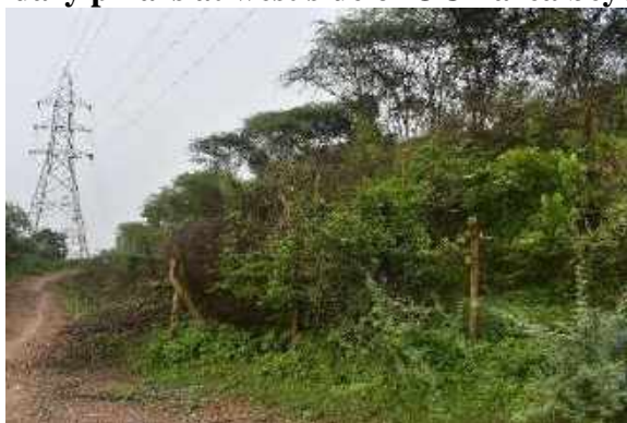
Plate 35: Safety zone demarcation and afforestation at west side (Dump-6 & 7) along Lilagarh Nala
