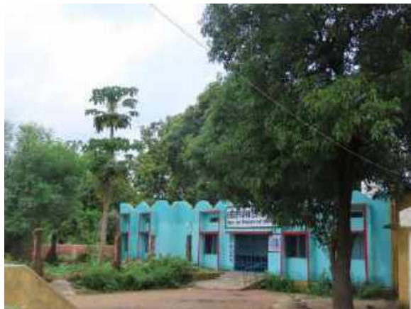
Construction of Adivasi Asharam at Udana
