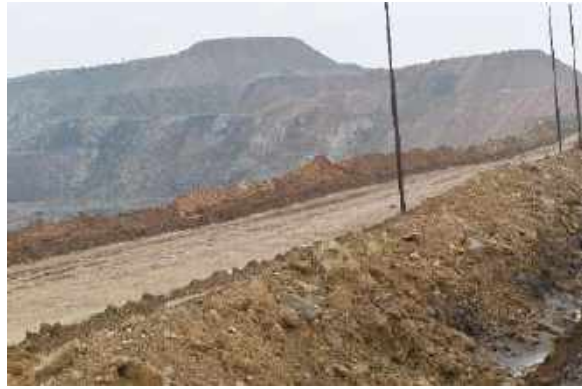
Catch Drain around quarry at east side along Hardibazar road
