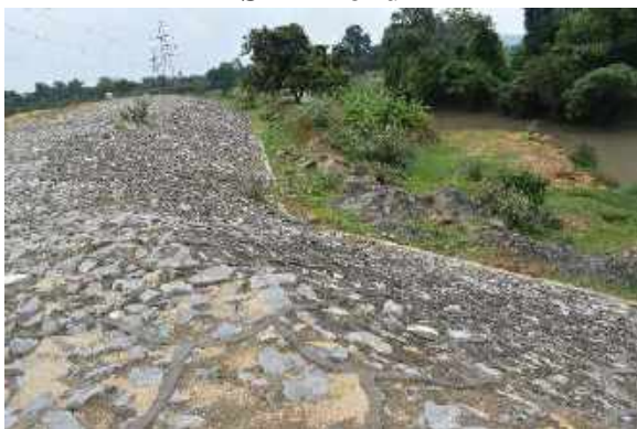
Embankment made alongside the Lilagrah Nala at quarry boundary
