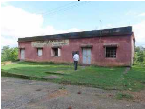
Construction of community hall around the project site
