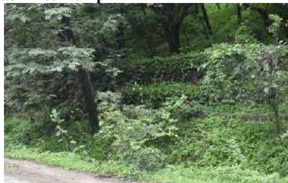
Gabion retaining wall for waste dump
