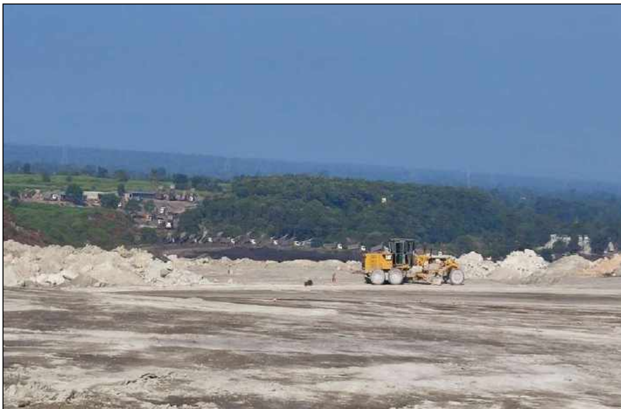
Photograph – 19: Backfilling in Chhal Opencast Project
