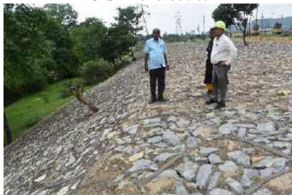
Embankment made alongside the Lilagrah Nala at quarry boundary
