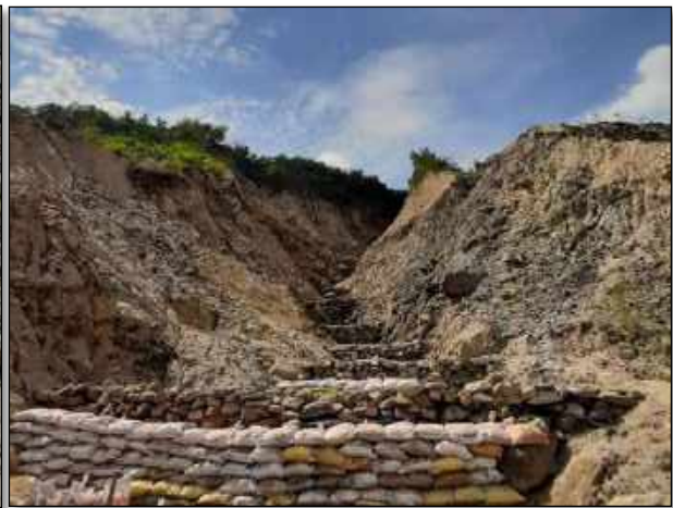
Fig 26: Check Dams to Arrest Soil Erosion
