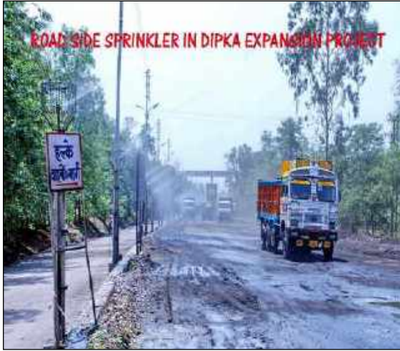
Fig 6: Fixed Sprinklers & Rain Guns for Dust Suppression at Coal Transportation Roads
