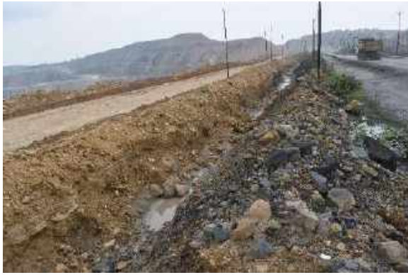
Catch Drain around quarry at east side along Hardibazar road
