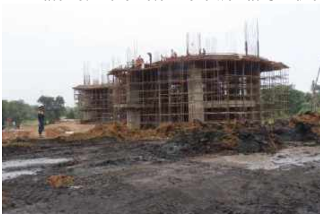
Plate 27: Silo under construction
