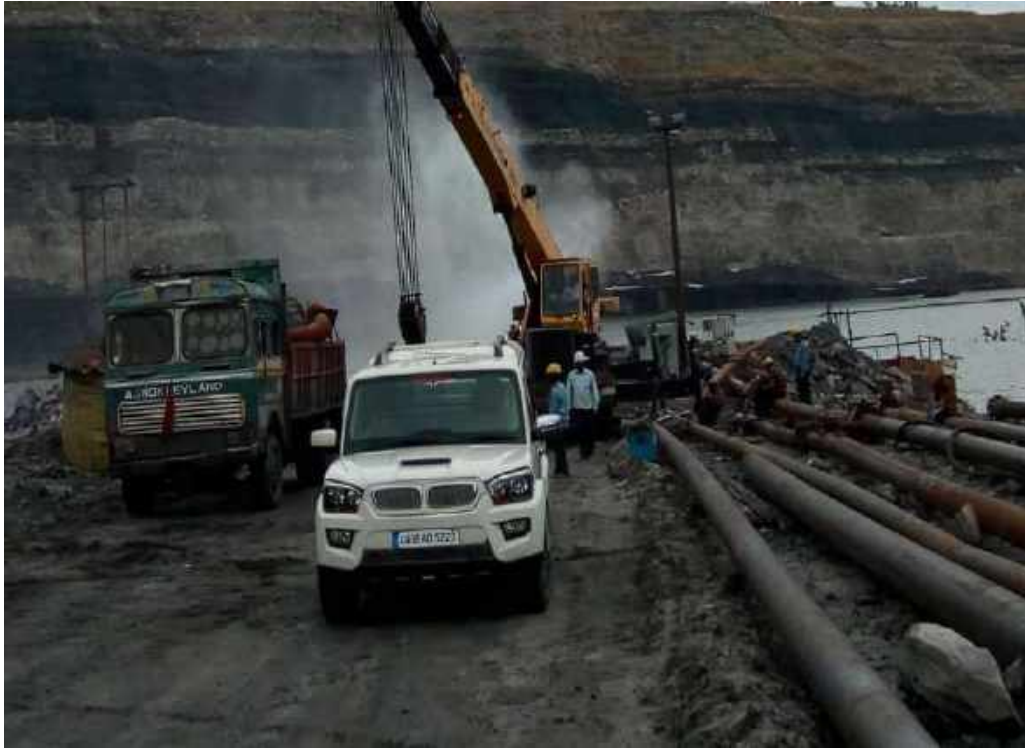
Fig.2.16 (B):- Water disposal system at the mine site.
