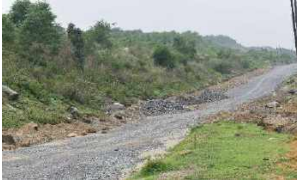
Eastern side slope of Dump-6 & 7
