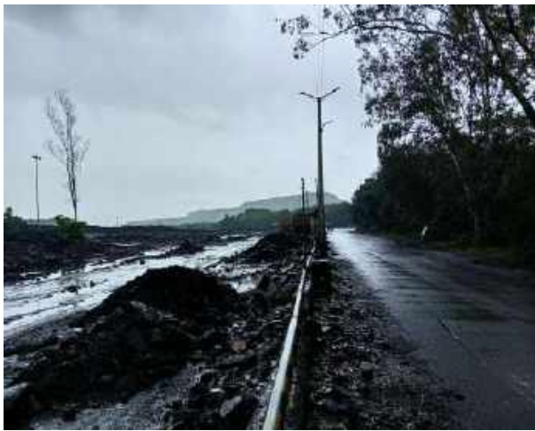
Plate 10: Fixed sprinkler along CT road with road condition
