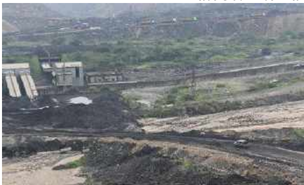
RCC retaining wall for TRS
