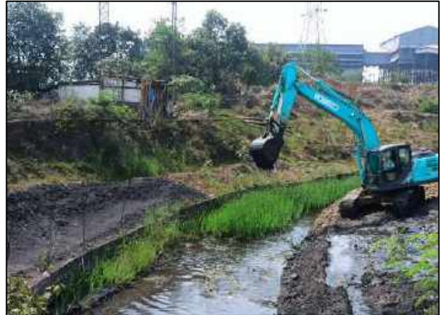
Fig 28: De-silting/Deepening and cleaning of ponds and drains
