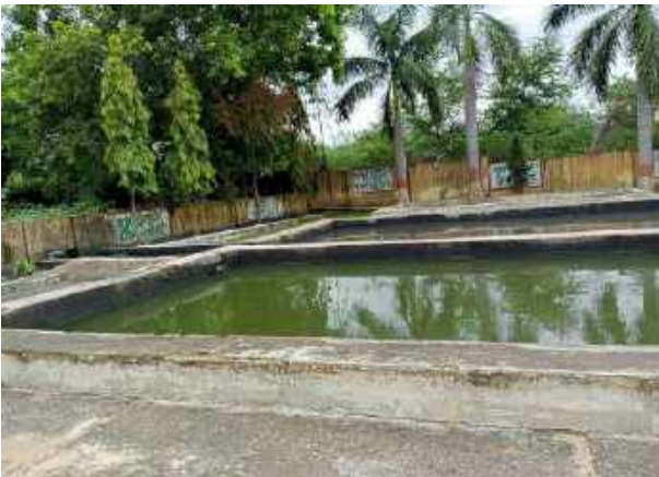
Plate 23: View of ETP with defunct Oil & Grease trap
