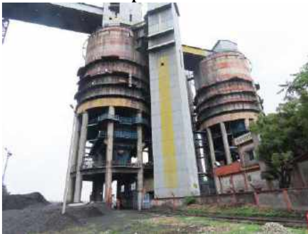
Plate 16: Silo with closed conveyor
