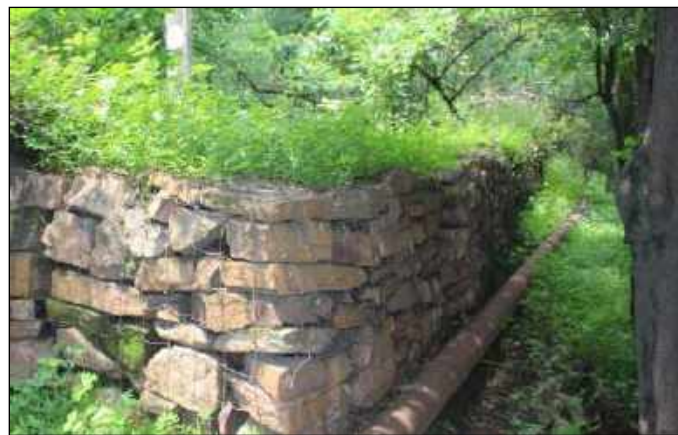
Fig 26: Check Dams to Arrest Soil Erosion
