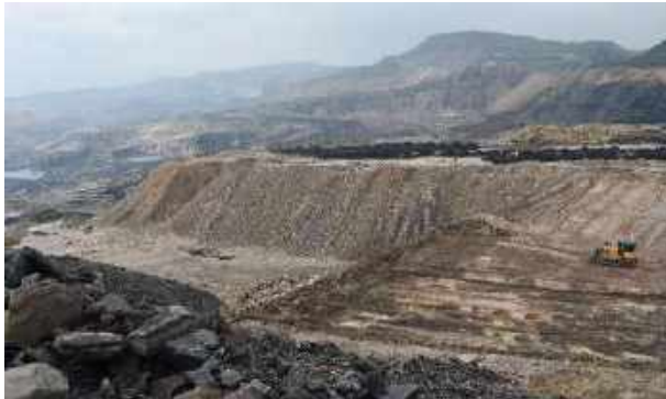
Internal backfilled dump towards northern side
