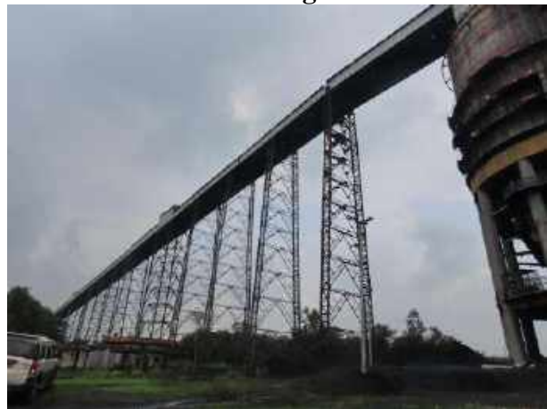
Plate 16: Silo with closed conveyor
