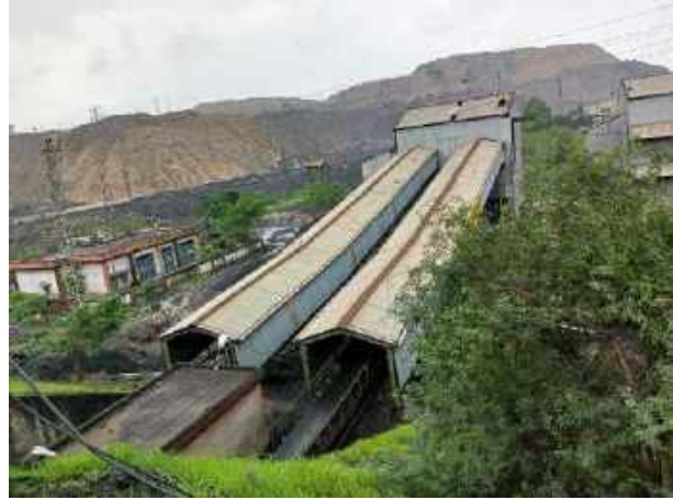
Plate 5: In pit close conveyor belt
