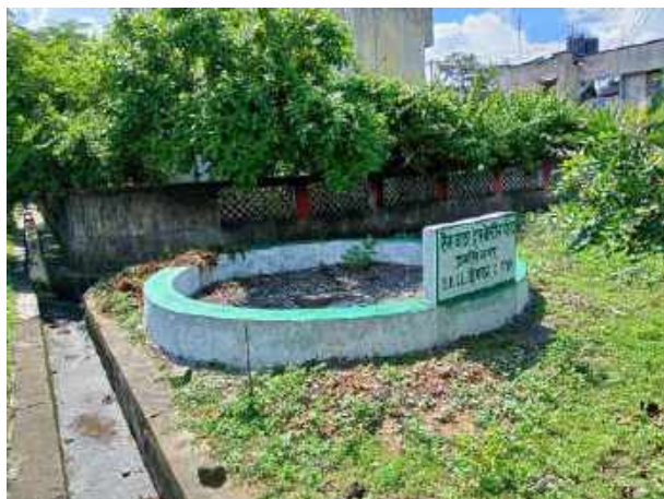
Plate 24: Rain water harvesting pit with open drain at Colony outside Quarter, Dipka OCP
