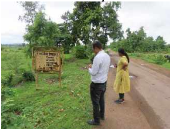
Butiminuous road from Baitari Chowk to Ranjhana Gram constructed under CSR activity
