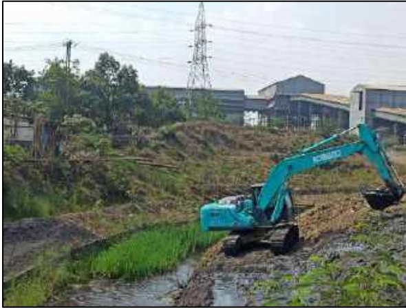
Fig 28: De-silting/Deepening and cleaning of ponds and drains
