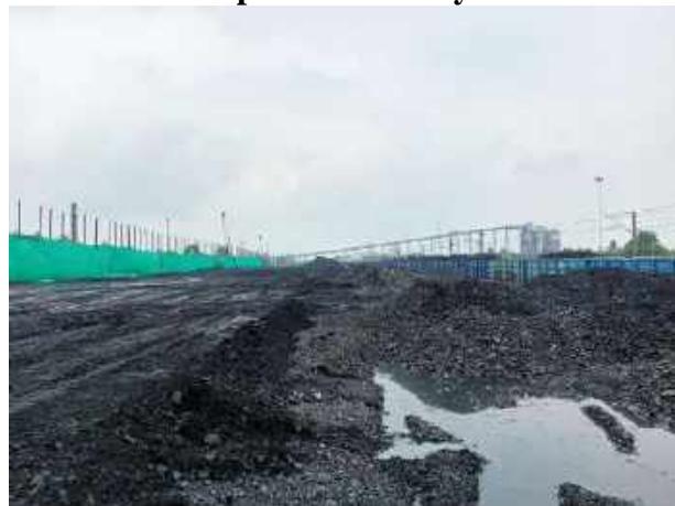
Plate 7: Wind barrier (net) at wharfwall of railway siding No. 2
