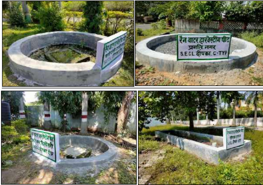
Fig 23: Rainwater Harvesting Structures
