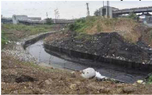
Drain provided for evacuation of excess surface water flow from N-NE to S-SW Plate 31 : Surface Water Management Structures
