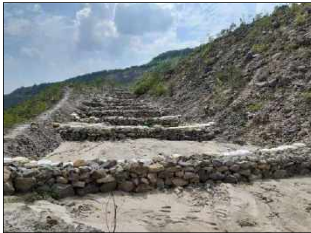
Fig 26: Check Dams to Arrest Soil Erosion
