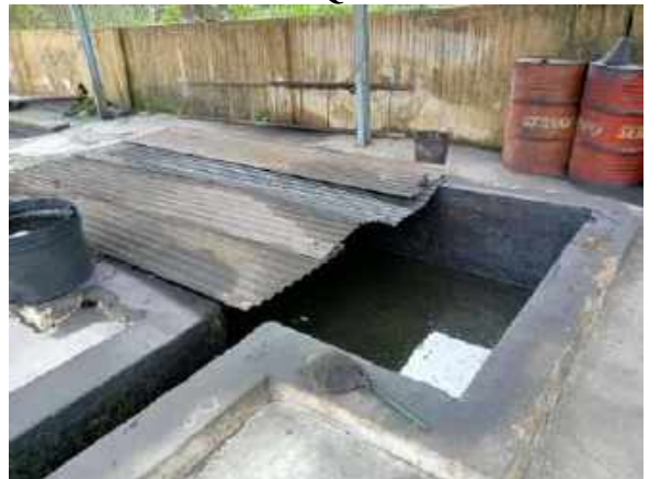
Plate 23: View of ETP with defunct Oil & Grease trap
