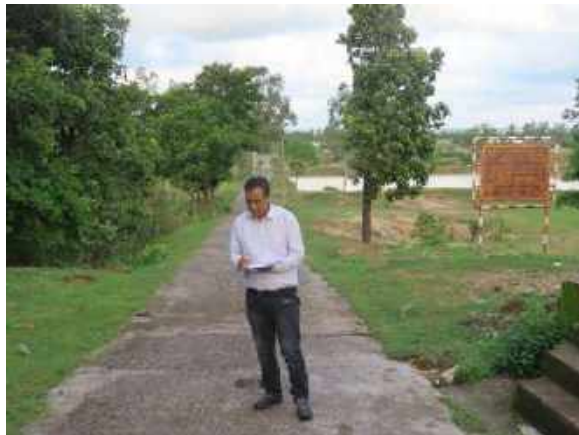
Construction of road, pond and beautification at Chodha Village
