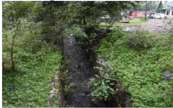
Drain provided for evacuation of excess surface water flow from N-NE to S-SW Plate 31 : Surface Water Management Structures
