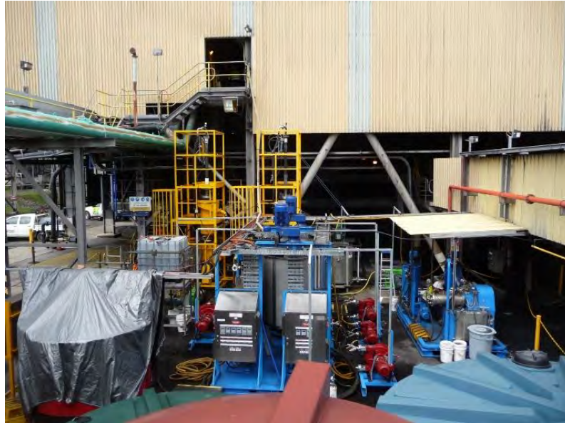
Fig. 3 The 3 t/day coal tailings treatment pilot-plant (Courtesy Glencore)
