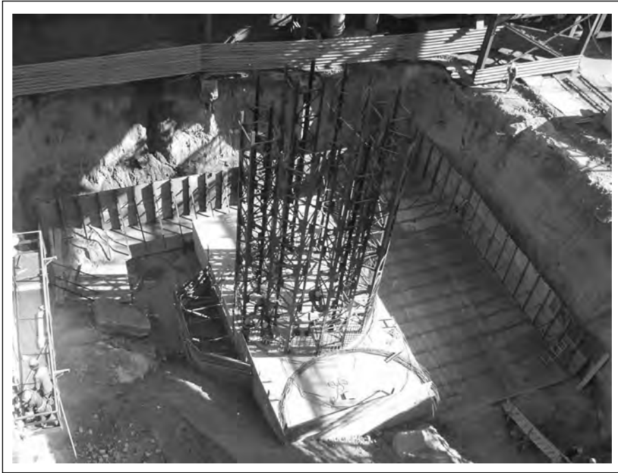
Figure 4: Erection of the Lead ISASMELT™ Furnace at UKMC
