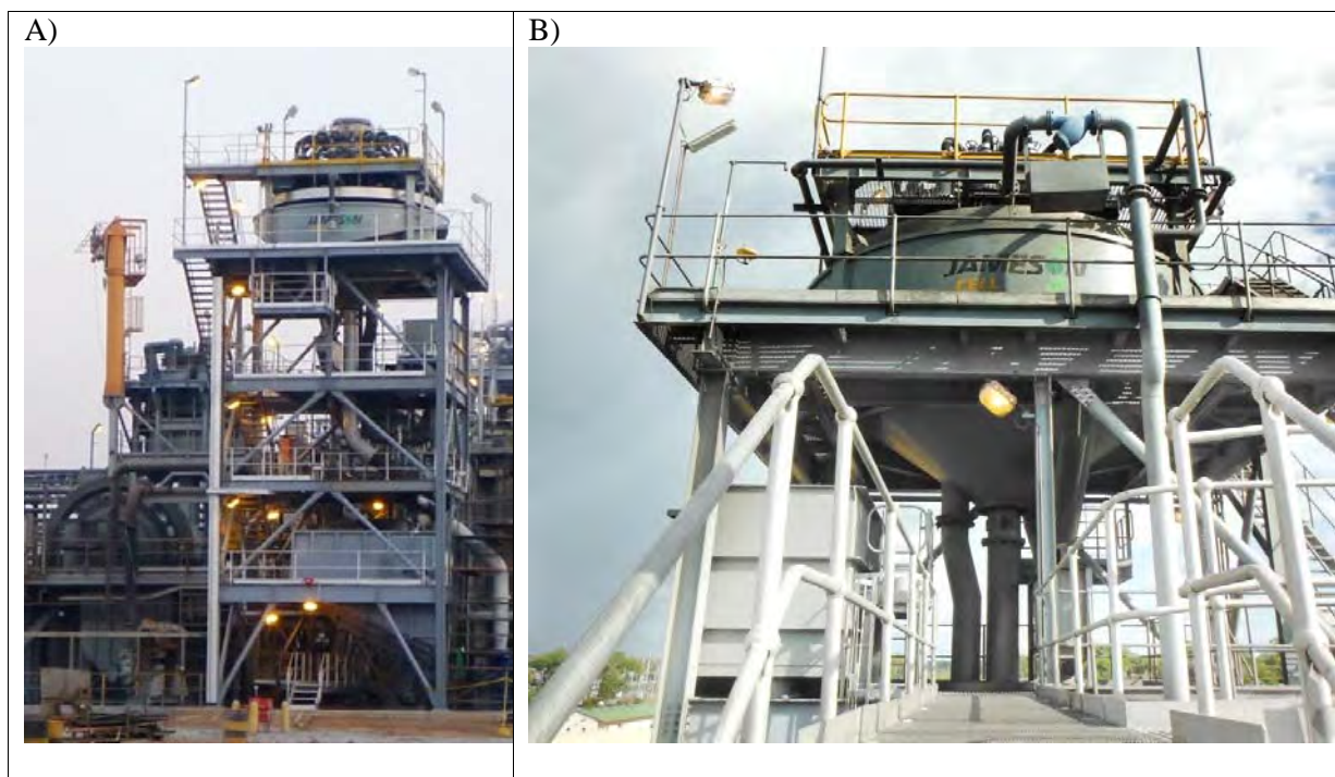
Figure 10 - The full scale model B5400/18 Jameson Cell installed at Lumwana
