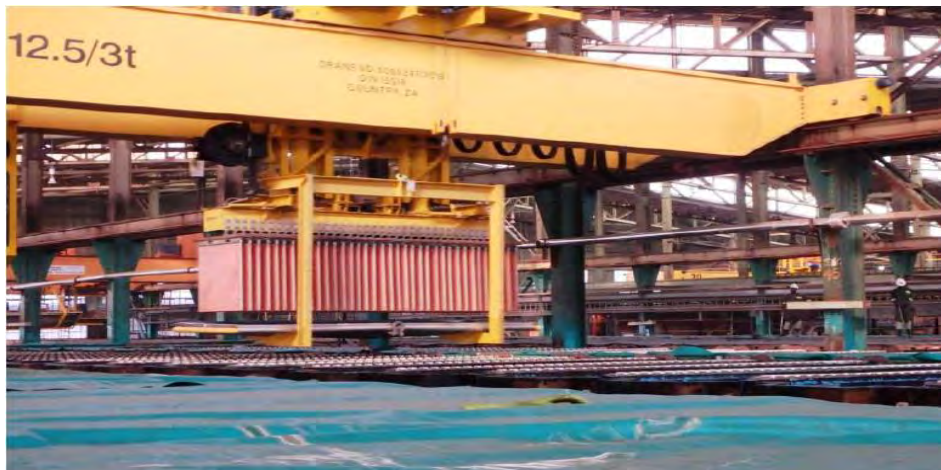
Figure 1. New overhead crane with drip tray carrying cathode plates.
