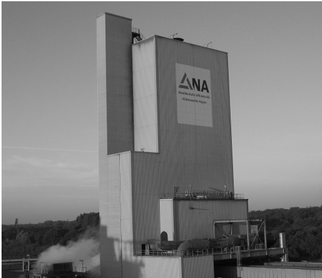
Figure 2 - ISASMELT™ Plant at NA in Lünen, Germany
