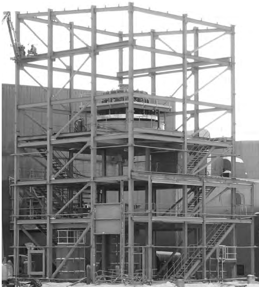
Figure 5: Construction of the new module for the Jameson Cell.
