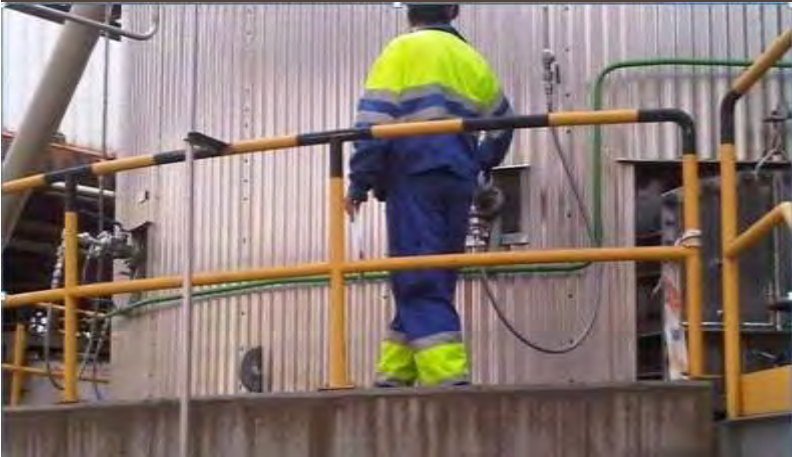
Oxidative Leach Circuit
