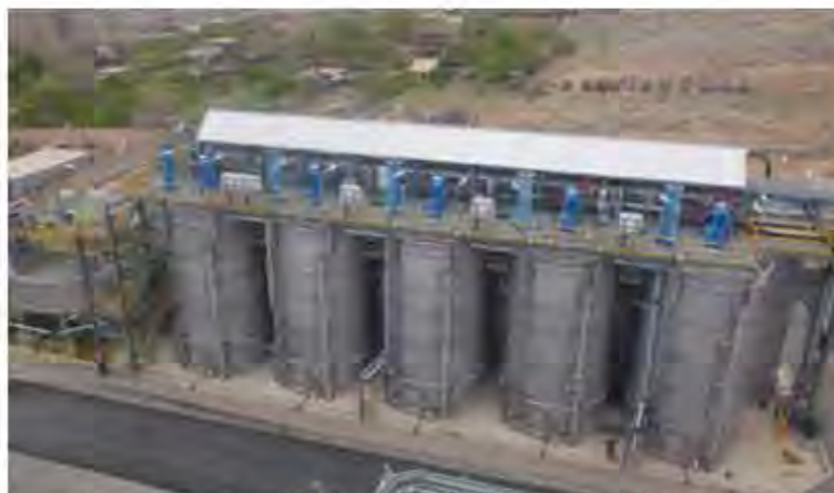
Figure 8 – The Albion Process oxidative leach plant in Armenia
