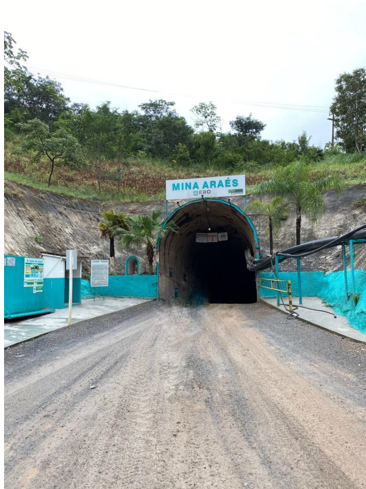
Figure 4 - Mine Portal (Xavantina, 2022)
