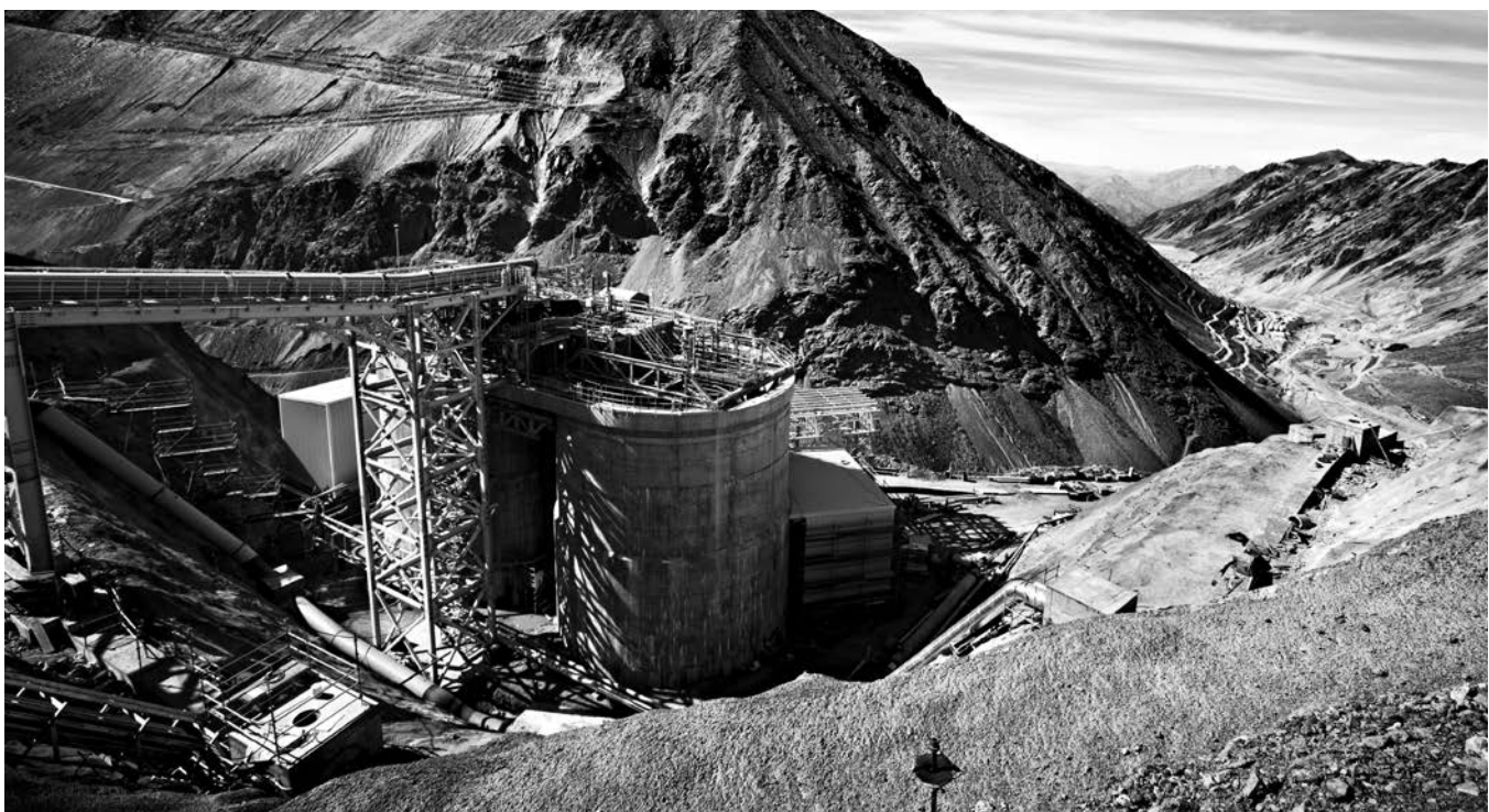
Holding tanks at the Confluencia plant at the Los Bronces operation in Chile.
