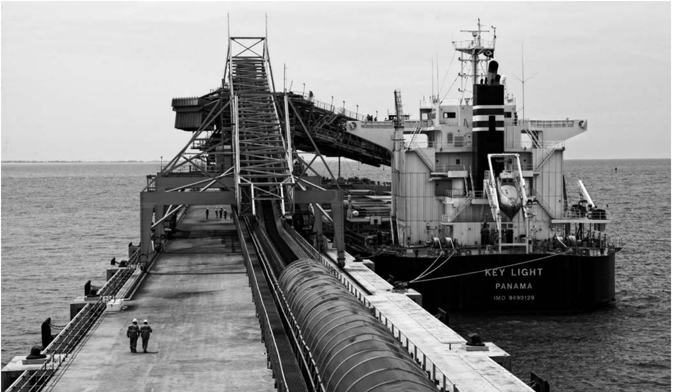
Loading iron ore from Minas-Rio at the dedicated export terminal at the Port of Açú in Brazil.
