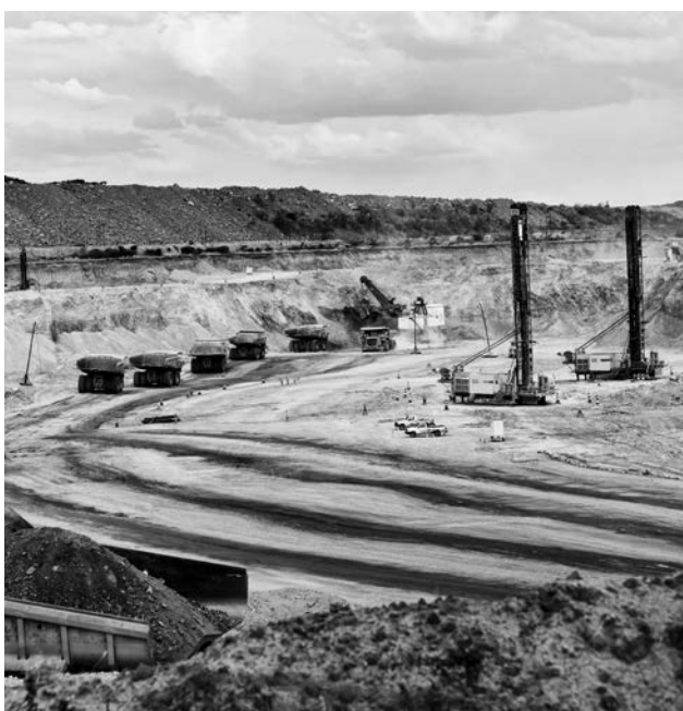
Drilling, loading and hauling operations in Mogalakwena's huge open pit.
