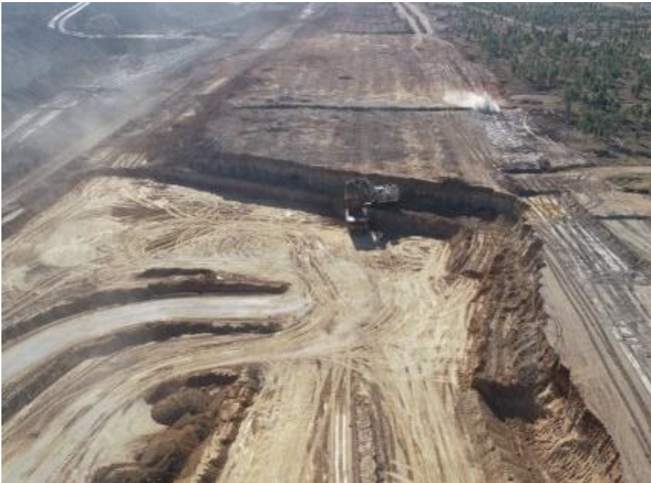
Tour of Capcoal's open cut operations
