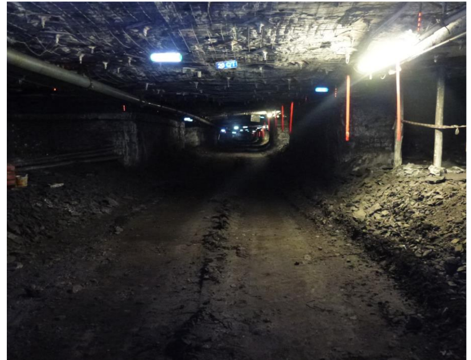
First development unit in place (above), with first coal cut late September 2019
