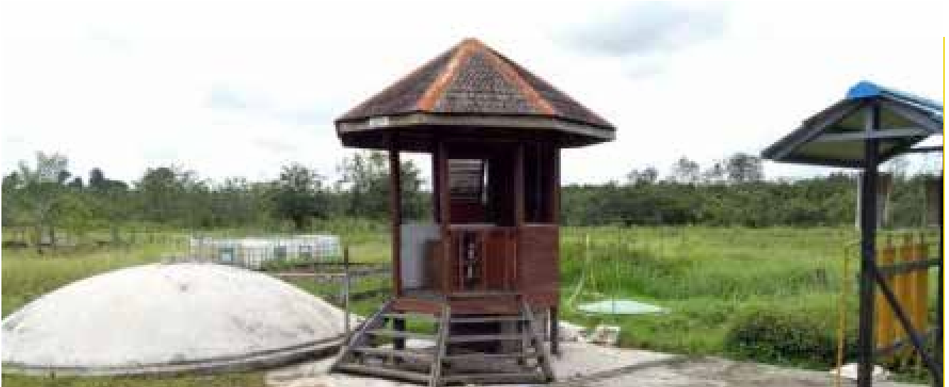
Pengembangan Fasilitas Bio Gas di PESAT (Peternakan Sapi Terpadu) Development of Biogas Facilities in PUSAT (Integrated Cattle Farming)
