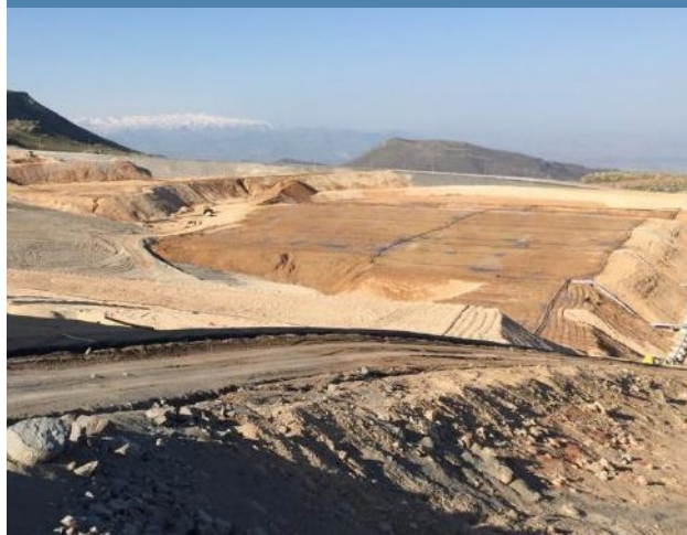
Stacked Ore on Heap Leach Pad
