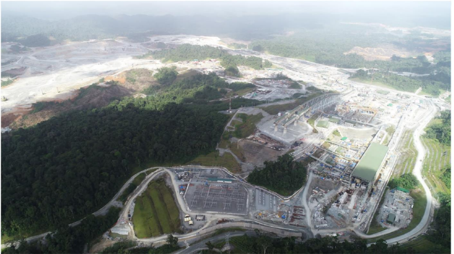
Figure 18-2 View looking SW over the Project processing plant, December 2018
