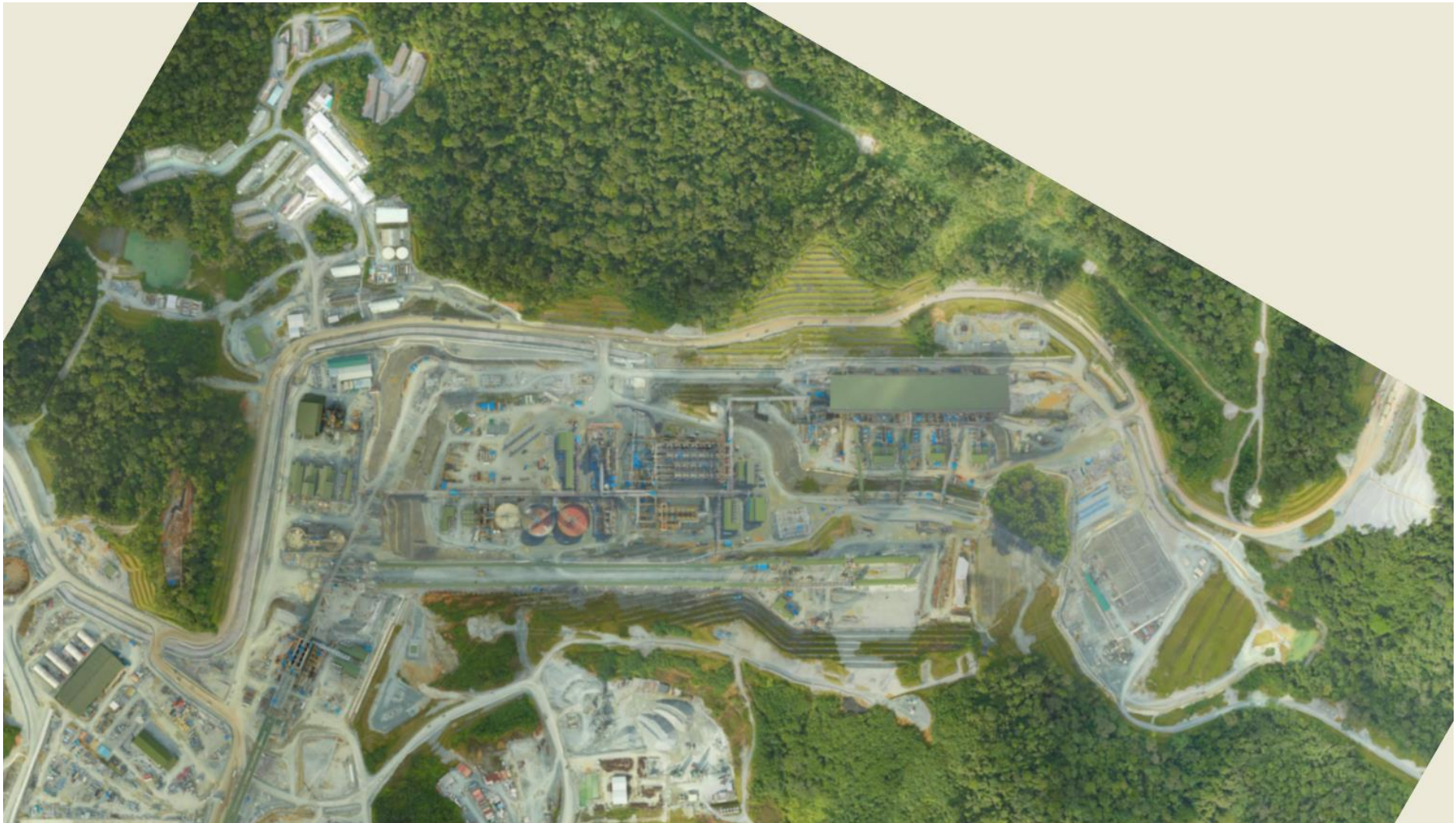
Figure 18-3 Photograph of as-built plant, December 2018
