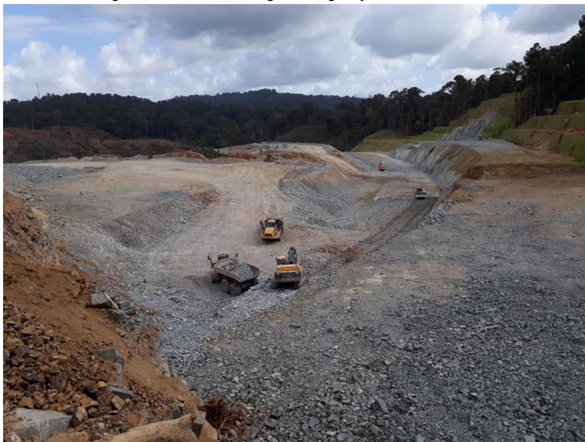
Figure 16-17 View looking east along Botija Pit diversion channel
