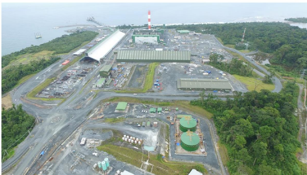
Figure 18-7 View looking over the port site and power station
