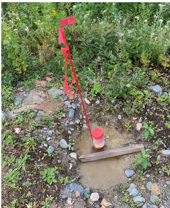
Figure 10.2 – Drill hole casing on the Project (photo August 22, 2019)
