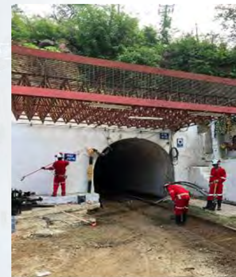
Tayoltita Portal and Rail Restoration
