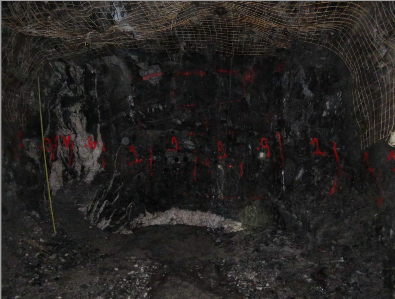
Figure 9.7 Level 2 East Round 8. Looking East.
