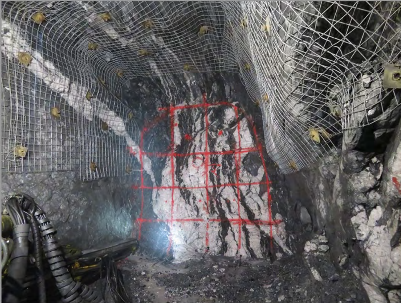
Figure 9.11 Level 3 East Round 2 (looking east)
