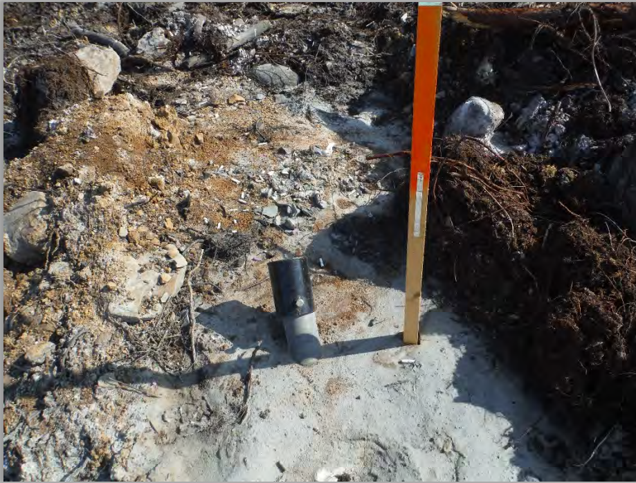
Figure 12.3 Historic Shaft Backfilled by NSDNR
