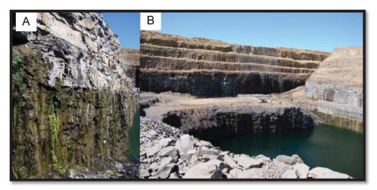
Plate 1: Mafutha Pitlake: Seepage through bedding plane fractures on the pit walls during lake filling (photo courtesy of Botha, 2012).
