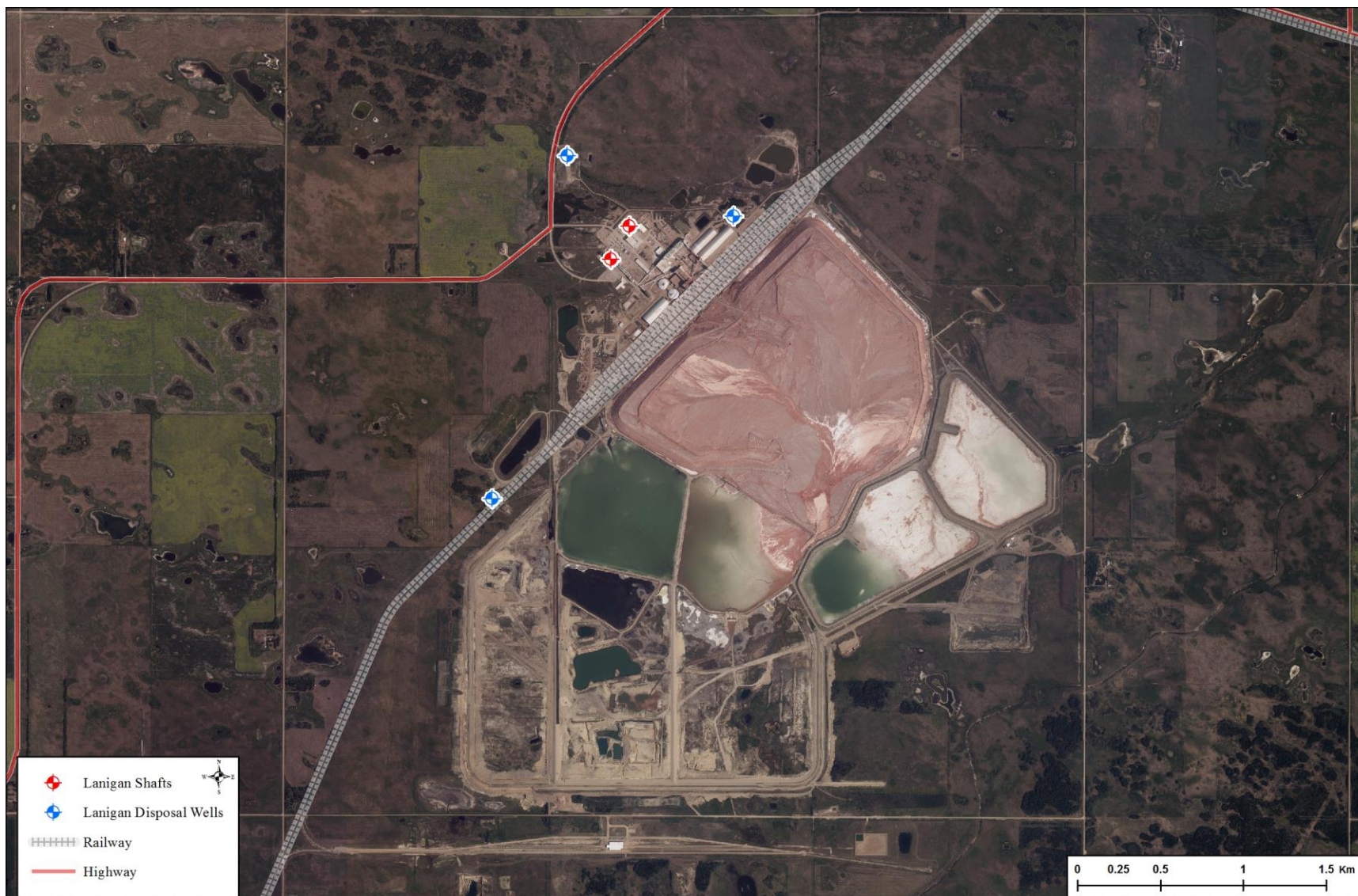
Figure 12: Air photo showing Lanigan Potash surface operations and Tailings Management Area.
