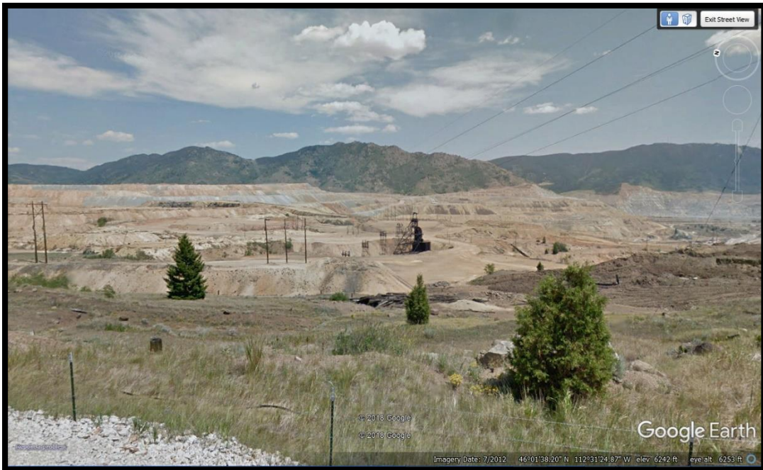
Figure 3.13-4 Views of North-South Embankment and Great Northern RDS from Granite Mountain Memorial via Google Street View.
