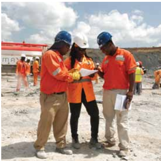
TONGON BLAST PREPARATION AT SZ PIT
