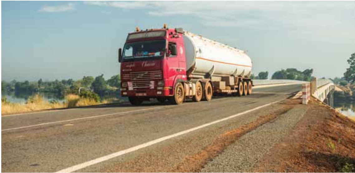
Infrastructure investments include new roads and bridges.
