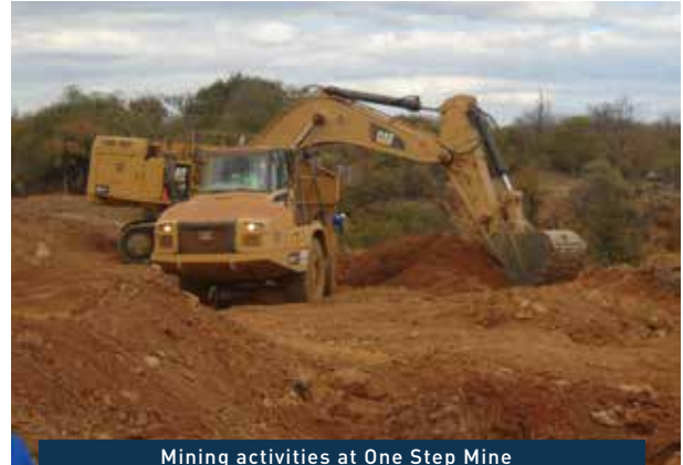
Mining activities at One Step Mine
