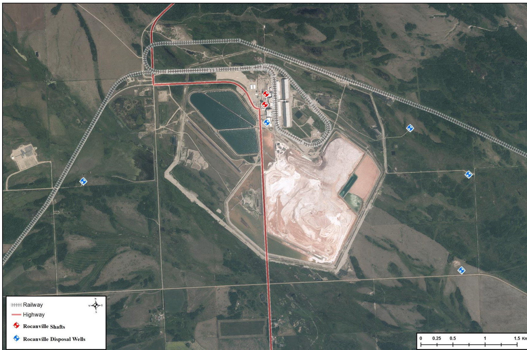
Figure 11: Air photo showing the Rocanville Mine surface operations and Tailings Management Area.
