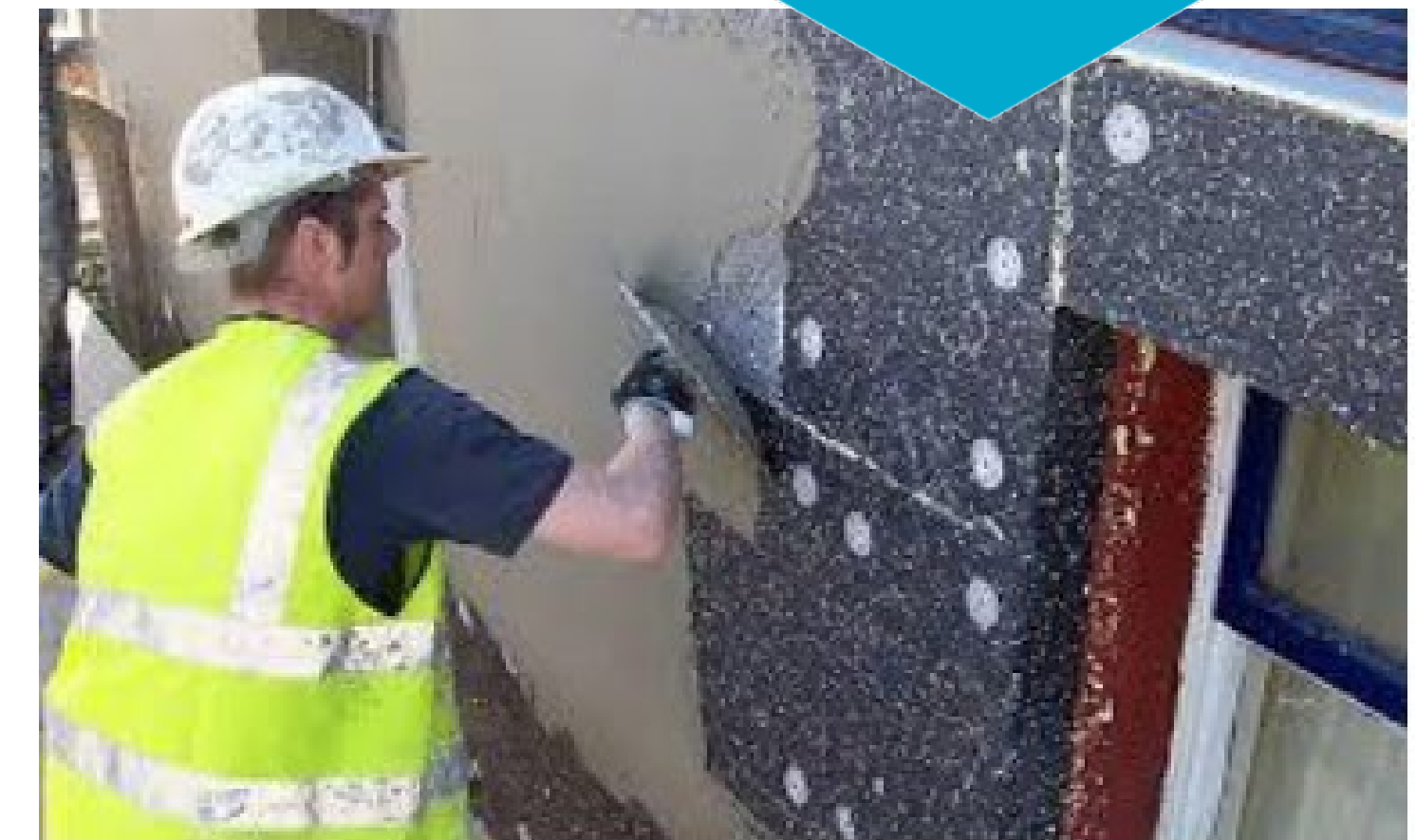
Installing Flame Retardant Foam
