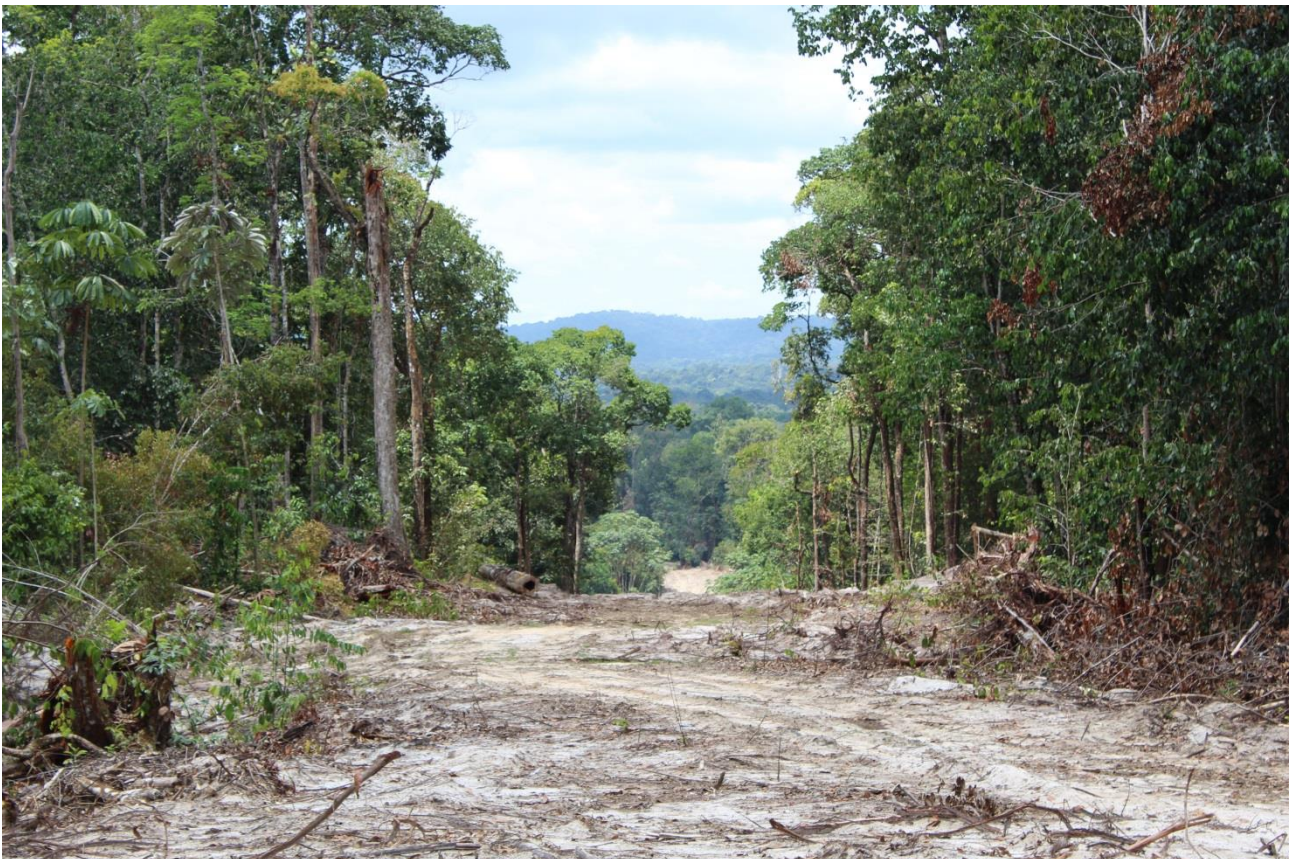
Figure 22: Access and haul road under construction
